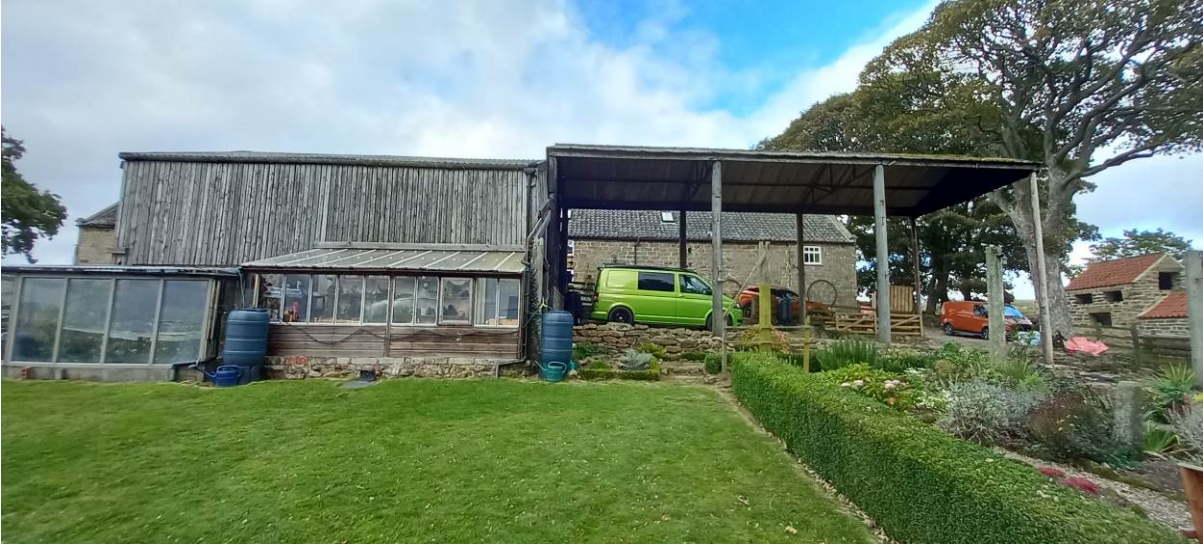
This photograph shows the rear elevation of the timber barn and pole barn to the south of the dwelling, and the siting of the proposed solar panels to the roof.
