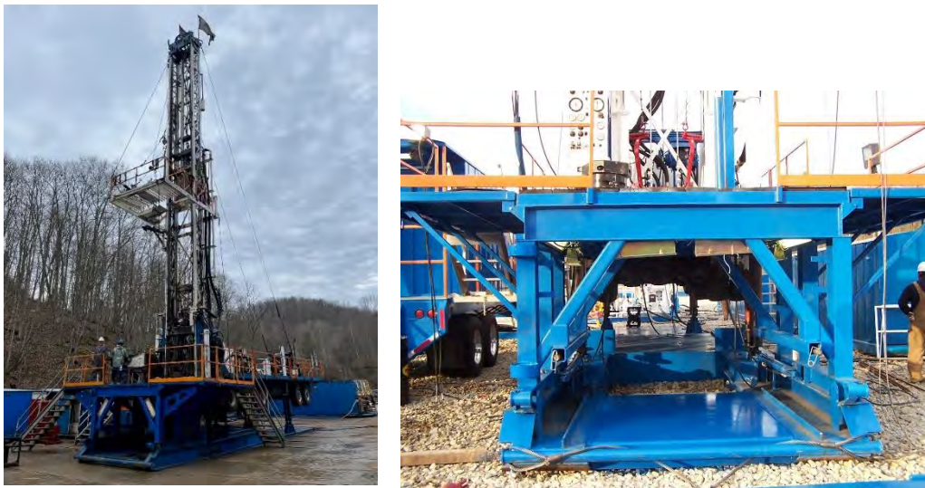
Image 3 – Speedstar Drilling Rig
