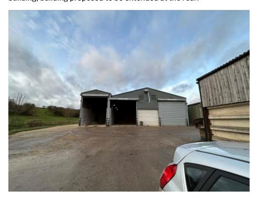
Photograph showing rear (north) elevation of existing agricultural grain storage building; building proposed to be extended on this elevation by 12 metres in materials and profile to match – existing fuel tank to be re-located north of extension.
