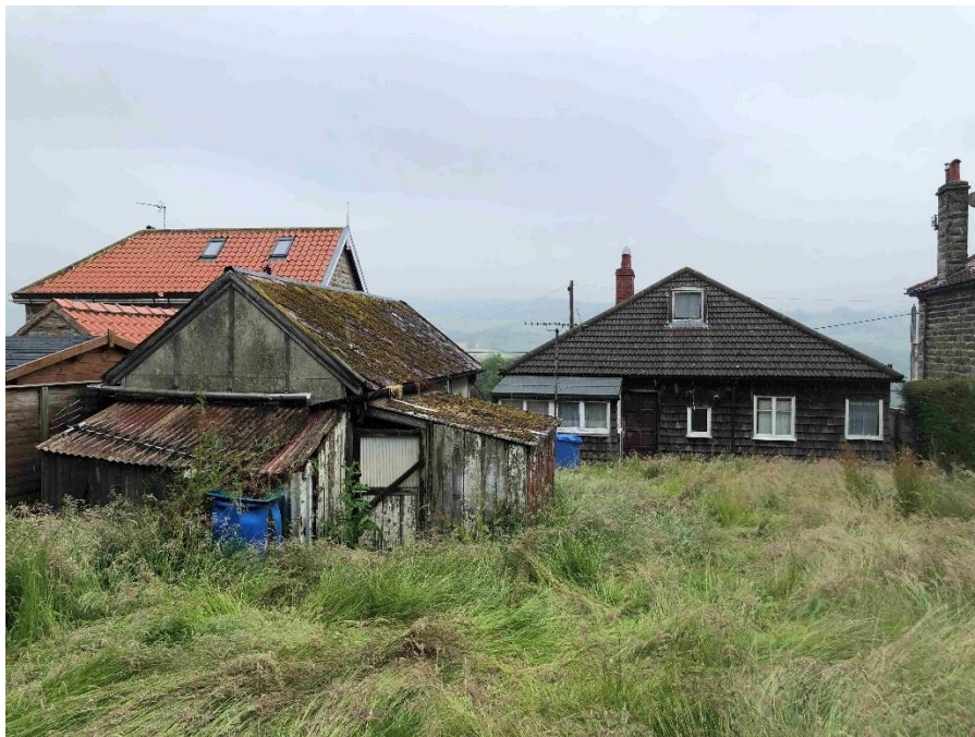
Photo 4 Rear elevation overview
