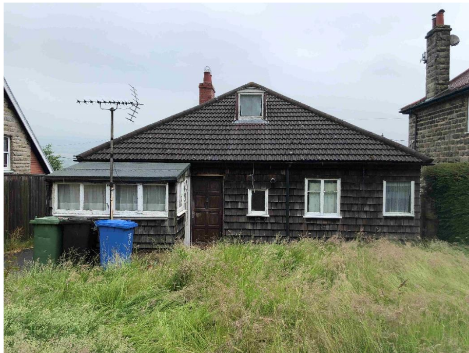
Photo 2 Rear (South) elevation
