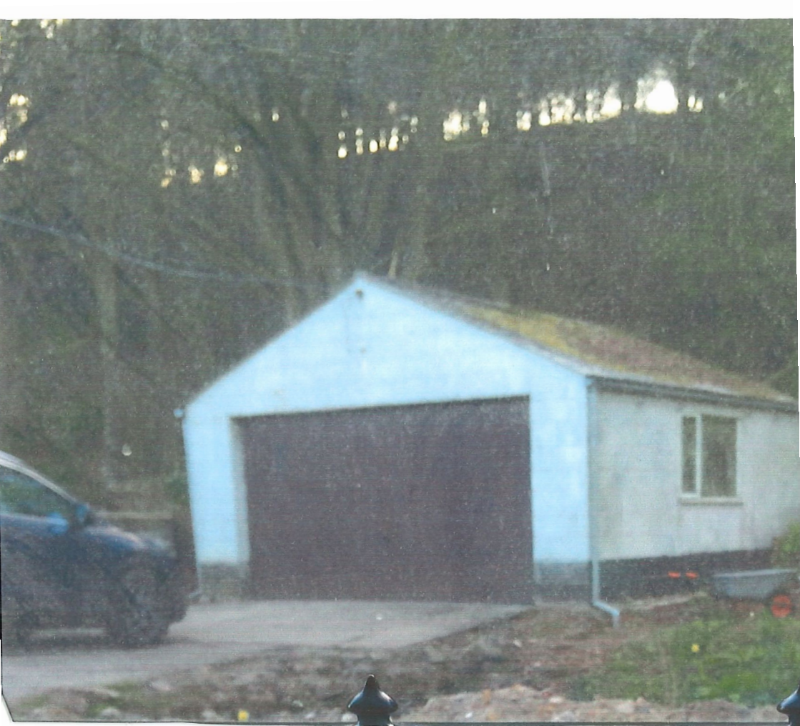
THIS IS WHAT THE OLD GARAGE LOOKED LIKE
