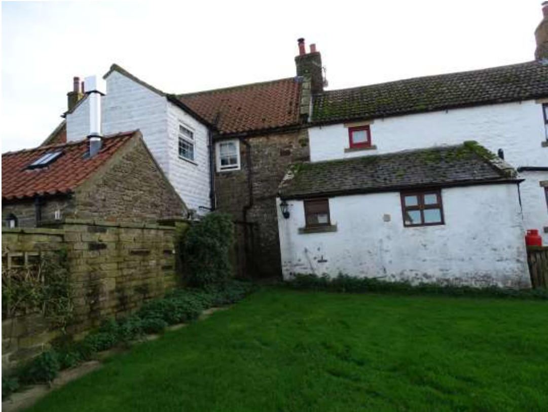
View of connection with neighbouring house. Note two storey rear extension to Listed house
