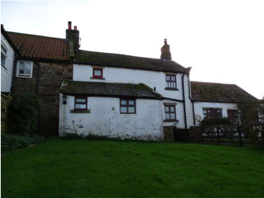
General view of rear elevation. Note garden level falls away and is lower than the internal floor level by between 30cm to 70cm.
