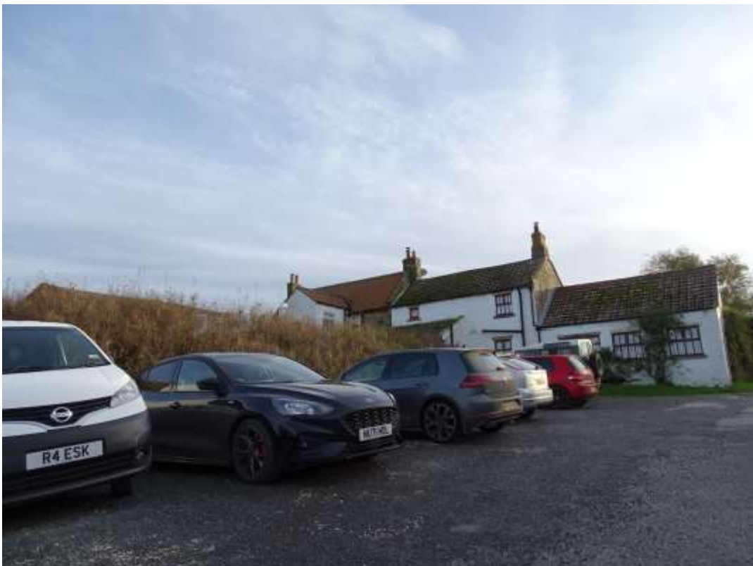
General view of the rear elevation and boundary against the commercial car park of Beacon Farm.
