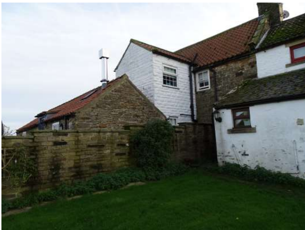
Stepped boundary with neighbouring house. Note substantial past extensions and conversion of outbuilding to neighbouring property of a substantial scale.
