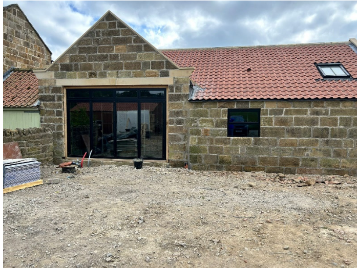
Roof as built
