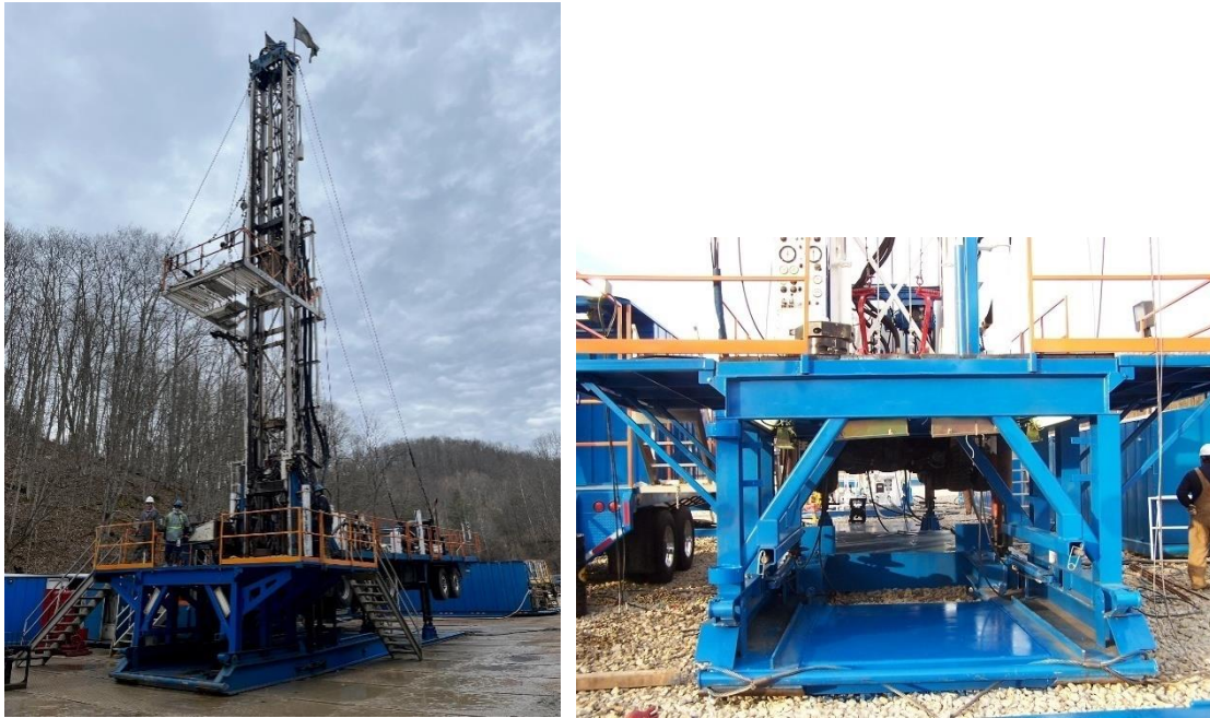
Image 3 – Speedstar Drilling Rig
