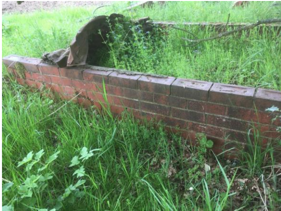
Fig 7. - Footings of the former building.
