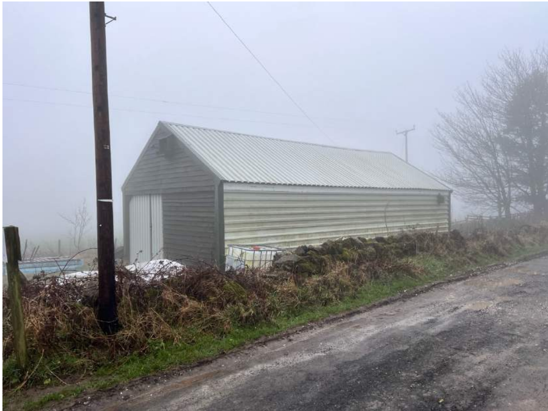
Photograph 5 – existing building adjacent to the application site
