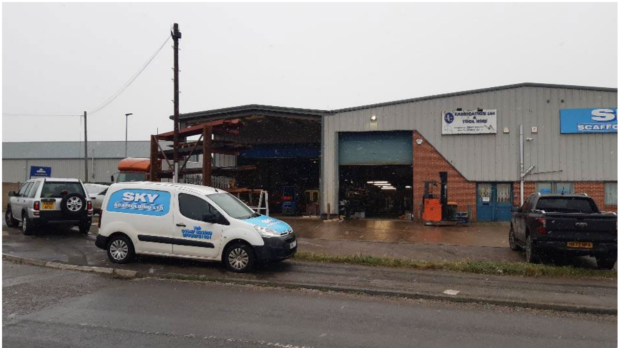
View of the unit from Farifield Way
