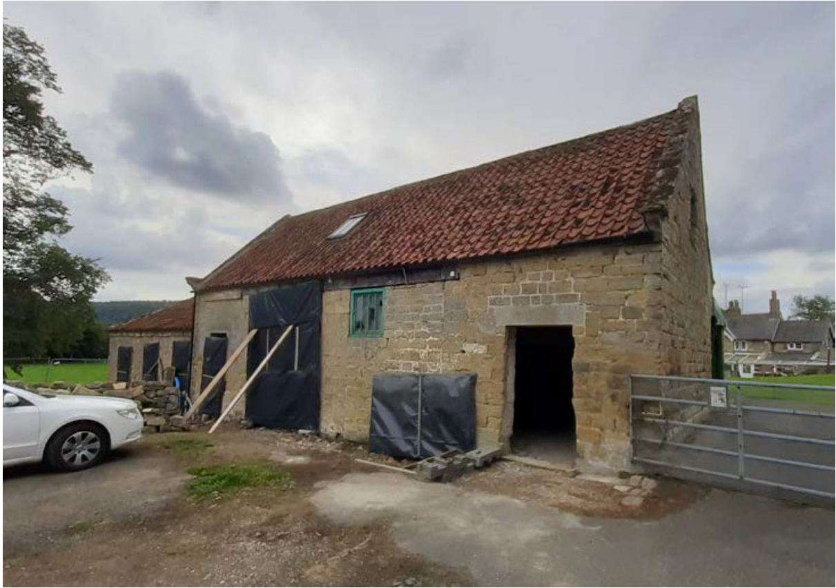
Front elevation of barn showing existing blocked up cart door opening to be re-opened
