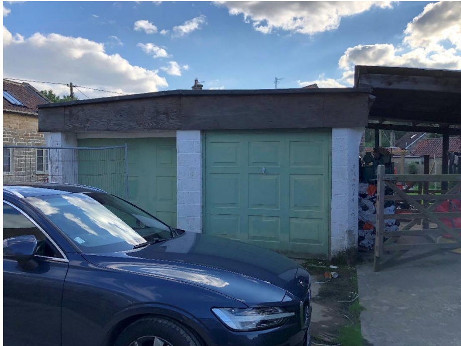
Part of the precast concrete building from the West
