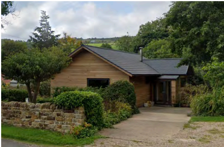
Fig. 6: View looking from the public highway (U2349) towards Wild Wood, a replacement dwelling using timber cladding and Envirotiles. Image credit: Google Streetview.
