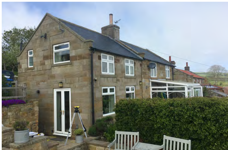
Fig. 24: View looking to the south-west corner of Quarry Cottage.
