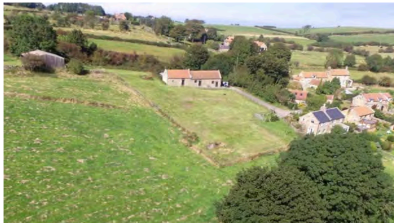
Fig. 4: Drone view from the south looking north with the slate roof of Quarry Cottage standing out against its neighbours. Image credit: Richardson & Smith Estate Agent.
