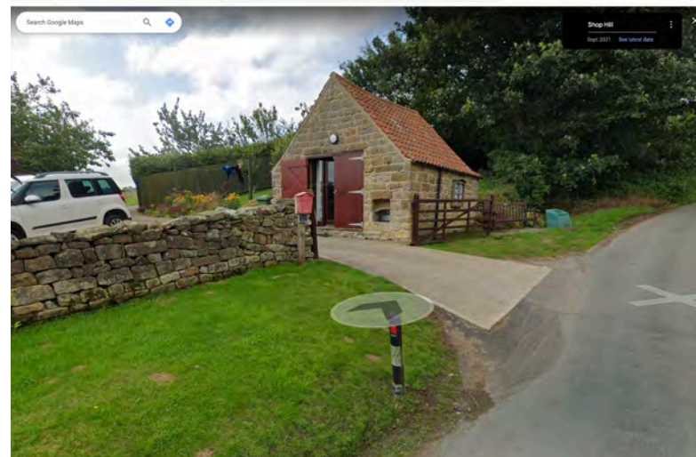
Fig. 9: View in 2021 looking from Shop Hill (U2349) towards the site access. Image credit: Google Streetview.
