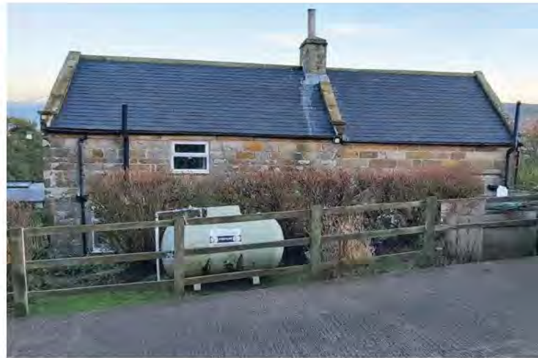
Fig. 18: View of the north-west elevation (rear) of Quarry Cottage from the drive. Image credit: Mr & Mrs Metters.
