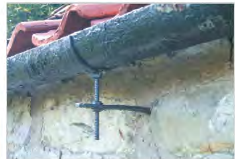
Painted rise and fall bracket supporting cast iron gutter (no fascia)
