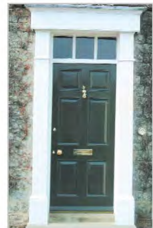
Georgian six-panel with surround and fanlight
