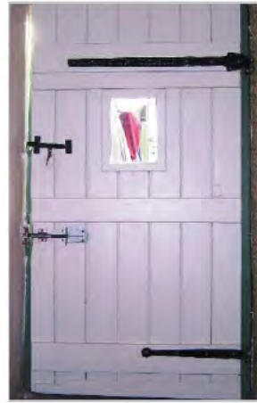
Ledged and boarded door with glazed panel and strap hinges
