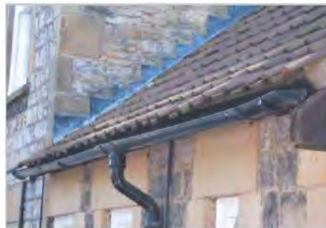
Half-round cast iron gutter (no fascia)
