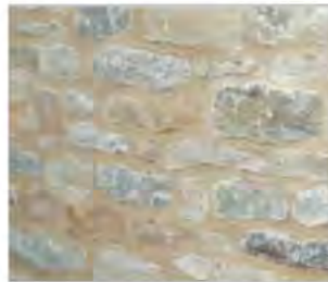
Bagged/ stippled pointing
