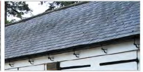
Gutter brackets
