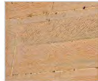
Ashlar stonework with fine lime-putty pointing
