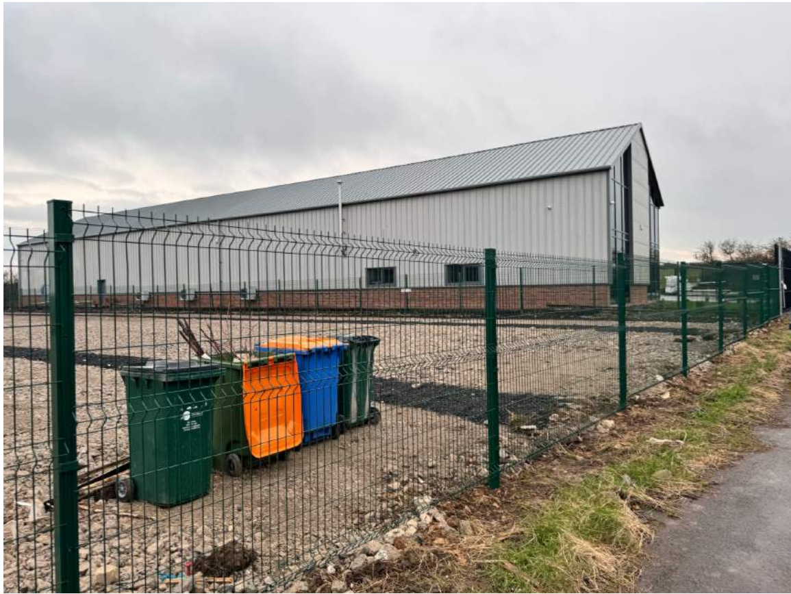
Photograph 2 - existing 2000mm steel fencing (retrospective)
