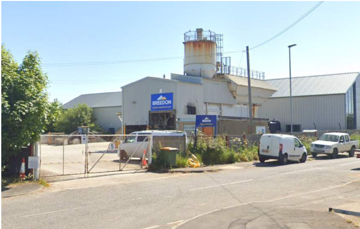
Photograph 3 - site prior to development (concrete plant)
