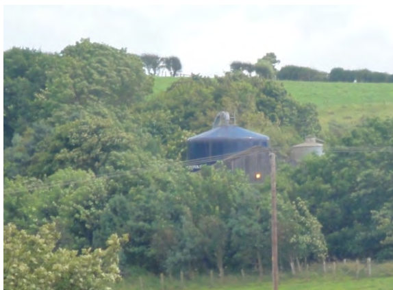
The visual impact of this silo is reduced by its location within a group of trees and its dark colour
