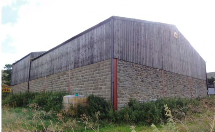
The use of stone helps to link the building to the more traditional buildings on the farm. A higher standard of material has been used on the most prominent elevation.
