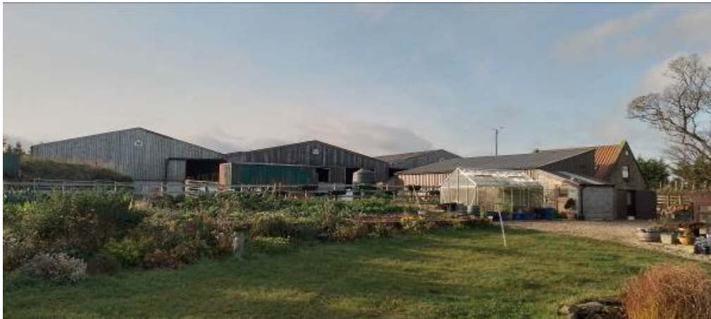
Building as already converted
