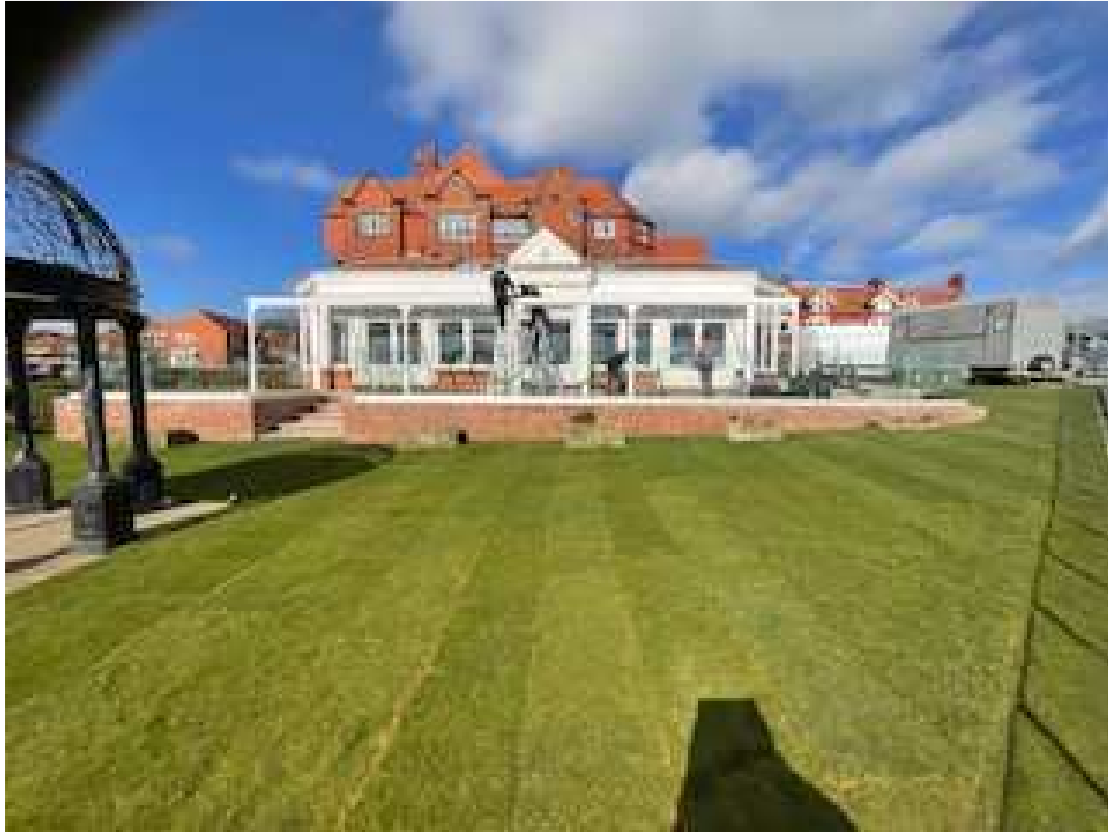
External view showing the glass balustrade to the external terrace and landscaped garden
