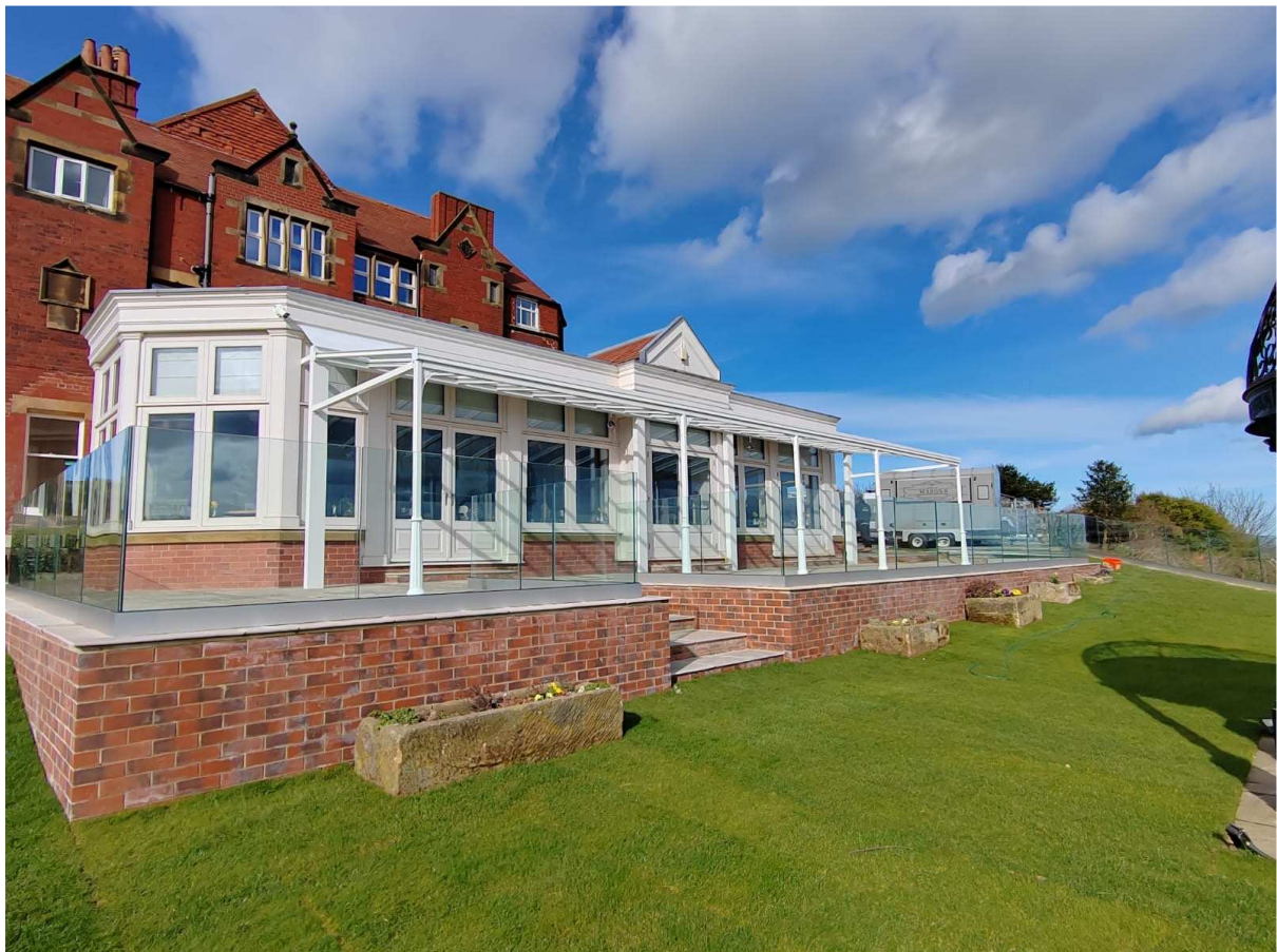
External view showing the canopy to the orangery and glass balustrade to the external terrace.
