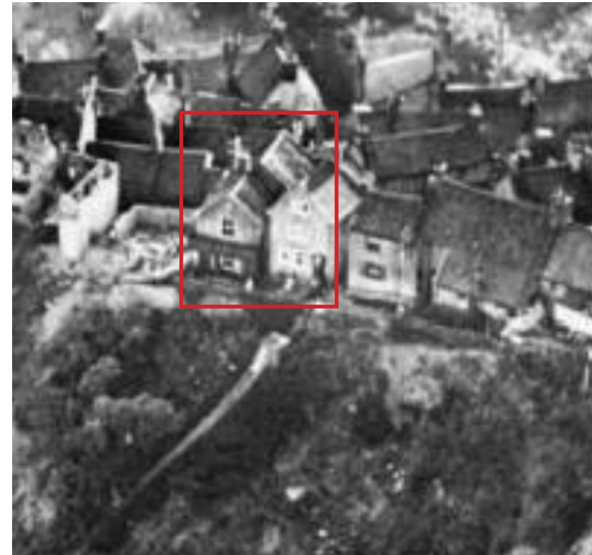
Image showing the loss of the adjoining house and rear extension to Cliff House
