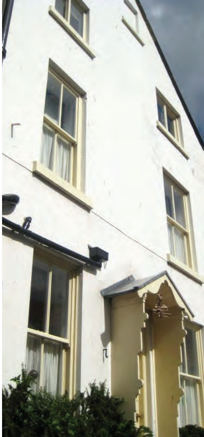
Cliff House in 2001 with the render still present.
