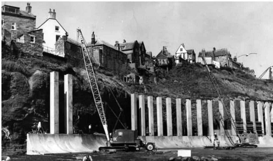
Construction of the sea wall in the 1970s
