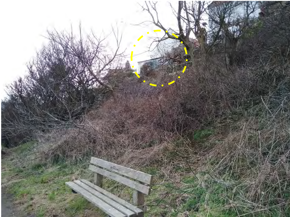
08 View from bottom of coastal slope looking towards the east elevation of Cliff House.
