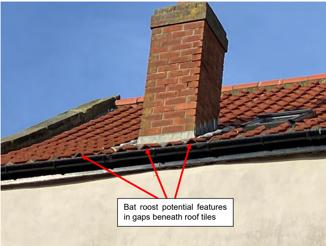
Photo 4. View of southern roof elevation.
