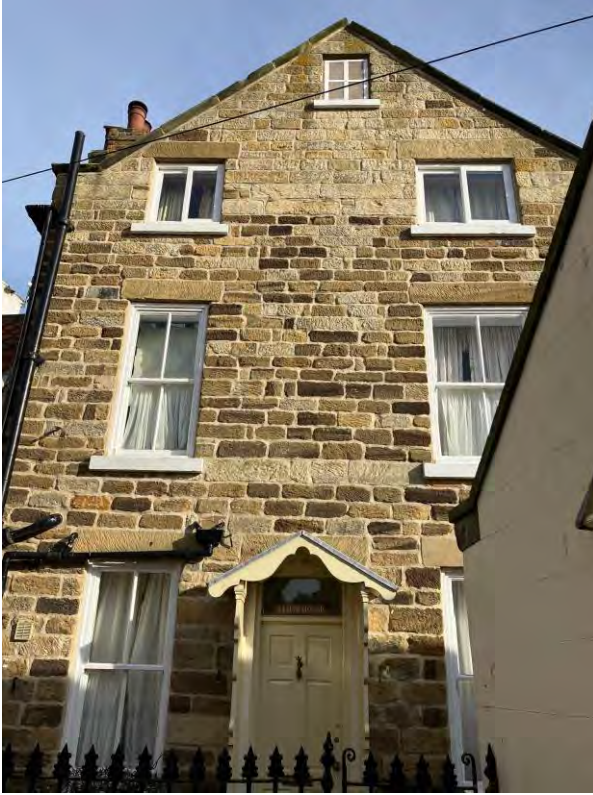
Photo 1. Western elevation of Cliff House – view looking east.
