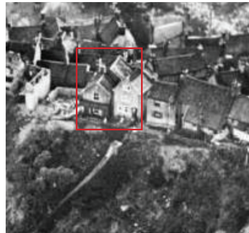
Image showing the loss of the adjoining house and rear extension to Cliff House
