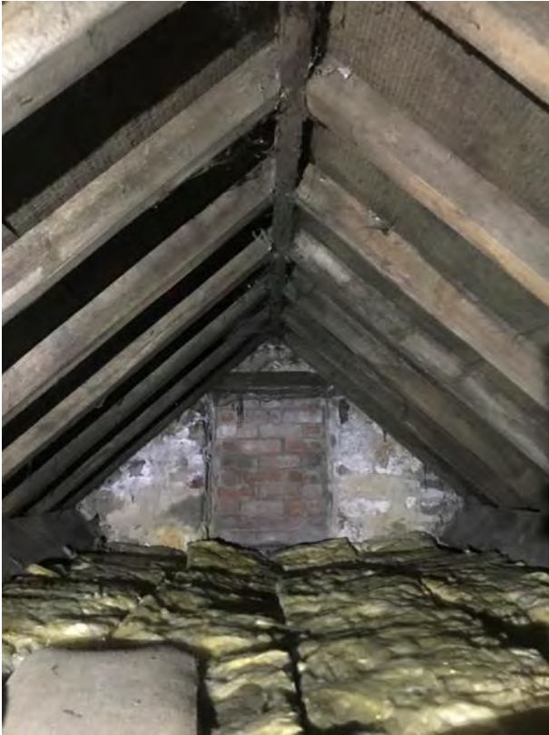
Photo 3. Cliff house internal loft space – view to western elevation.
