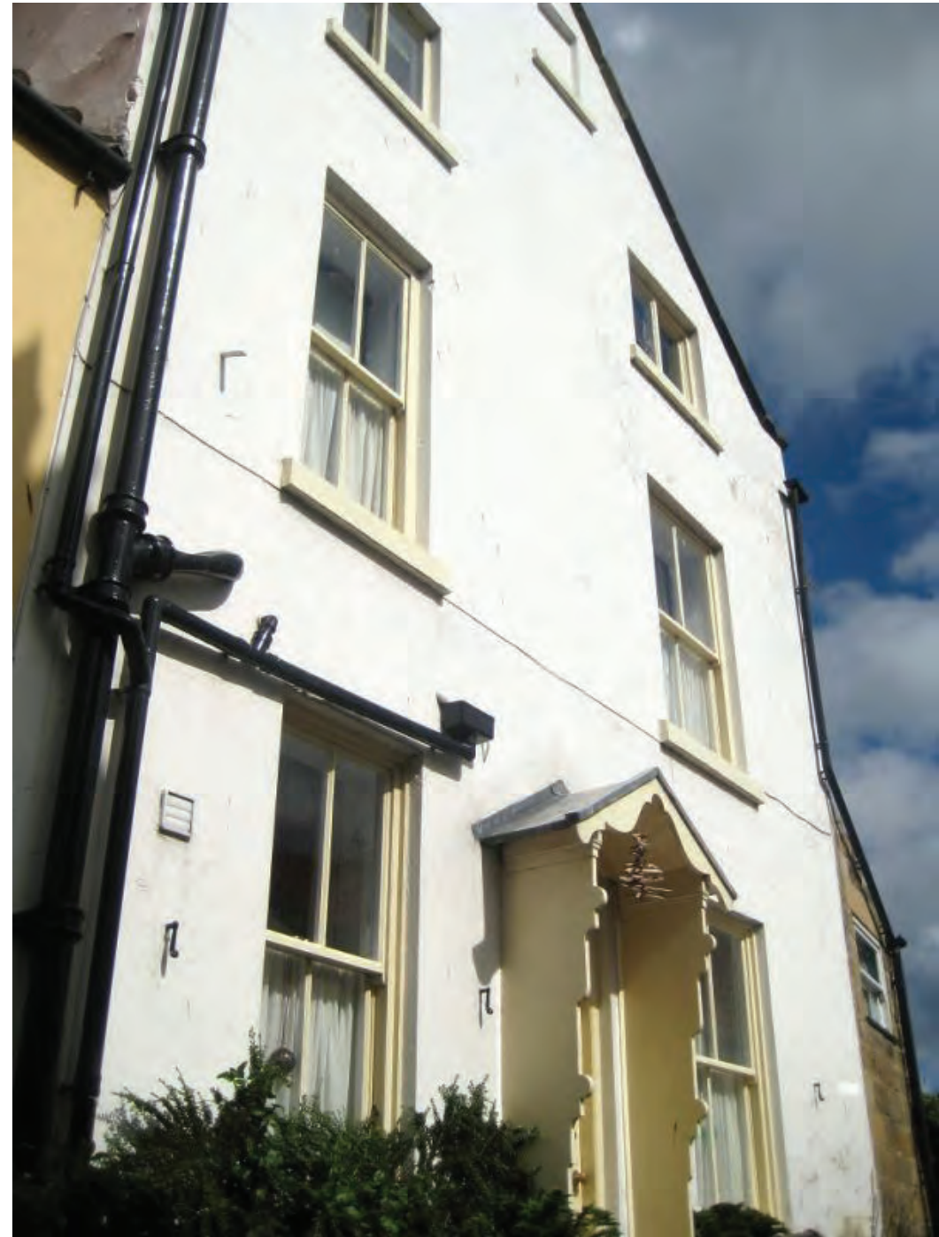
Cliff House in 2001 with the render still present.
