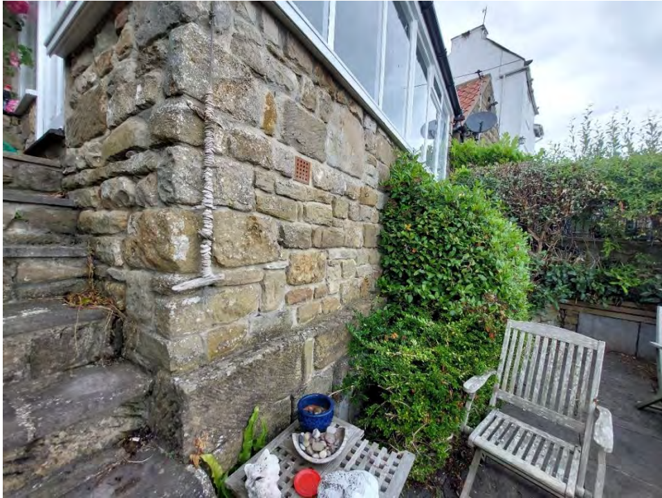
01 East elevation - view of the conservatory support wall and lower patio.
