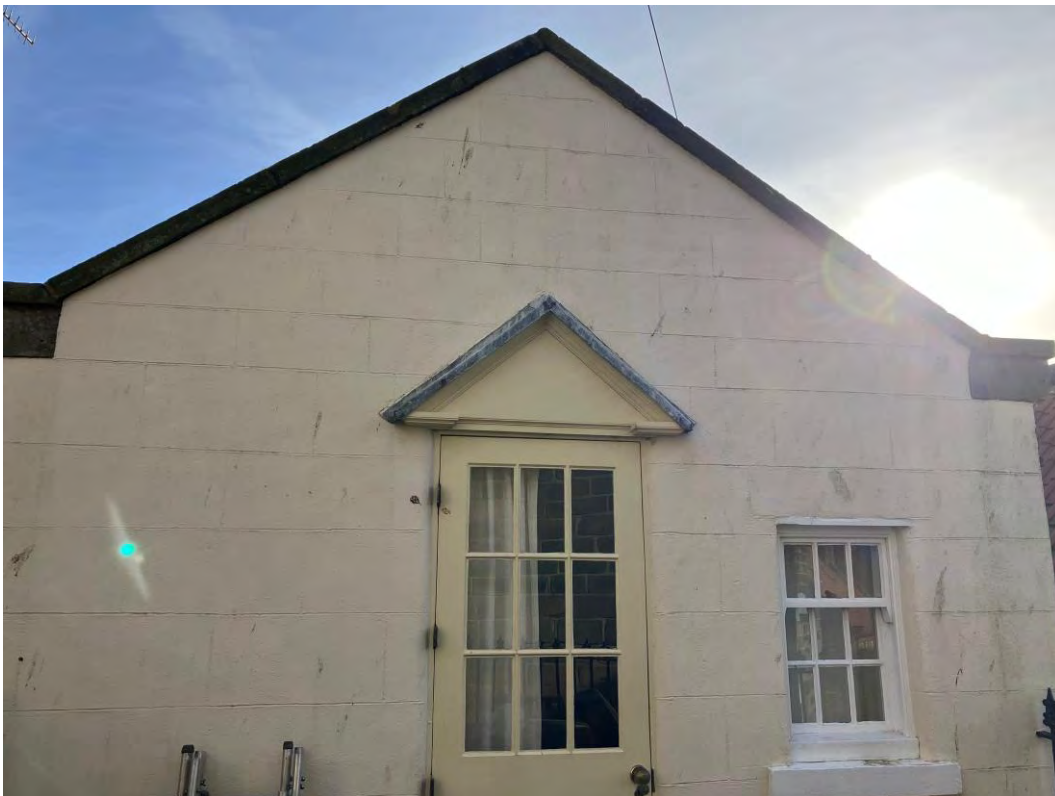
Photo 8. Northwest elevation of Annex building – view south.
