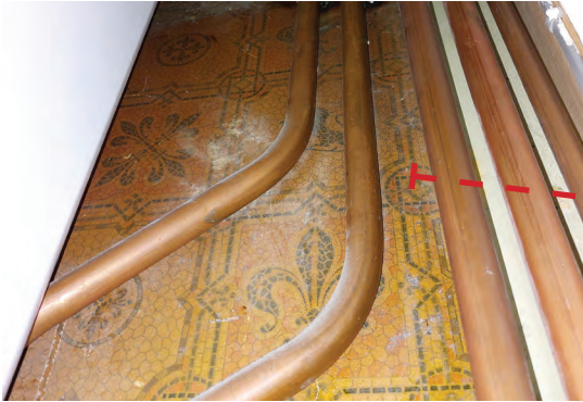
1900s wallpaper behind the hot water tank
