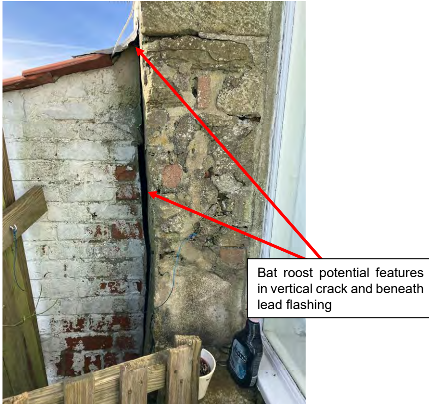
Photo 5. View of southern building extension adjoined to main building – view west.
