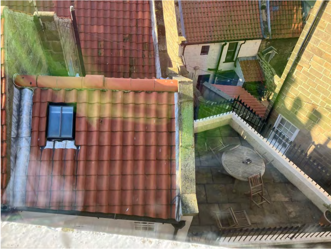
Photo 9. View of northeast roof elevation of Annex building.
