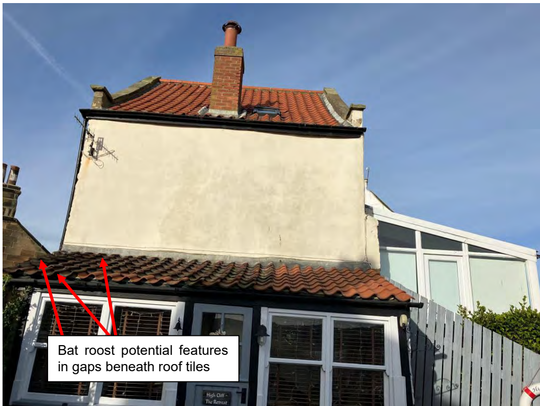
Photo 2. Eastern elevation of Cliff House – view west.
