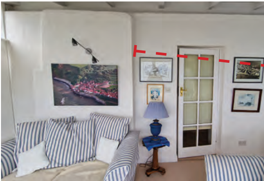
Chimney flue remains
