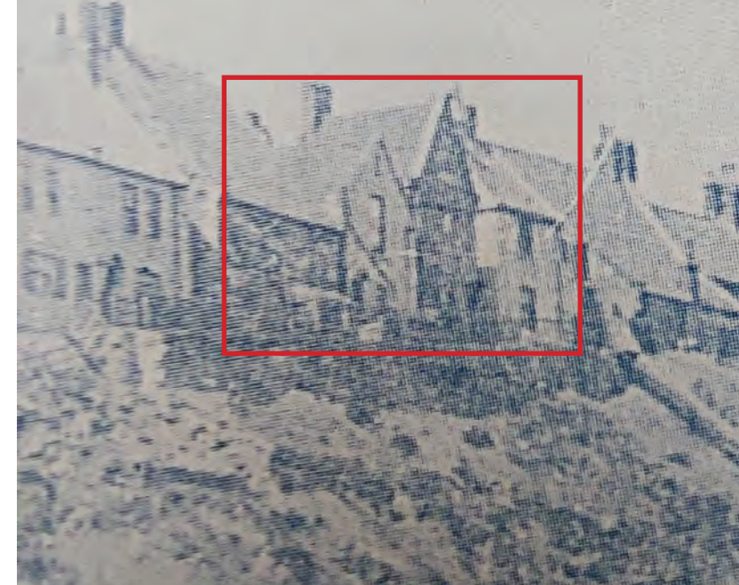
Image showing the house next door before being demolished and rear extension to Cliff House in 1891
