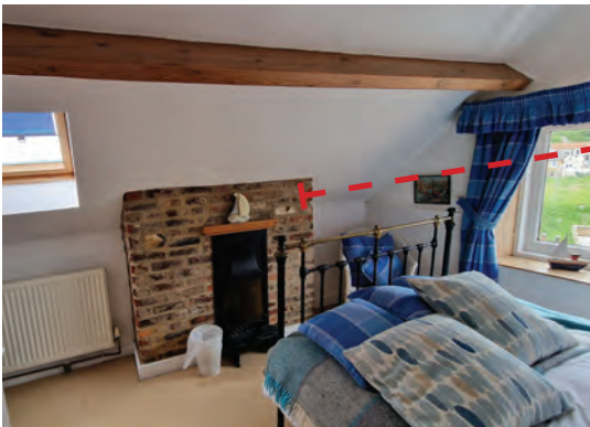
Fireplace to second floor bedroom
