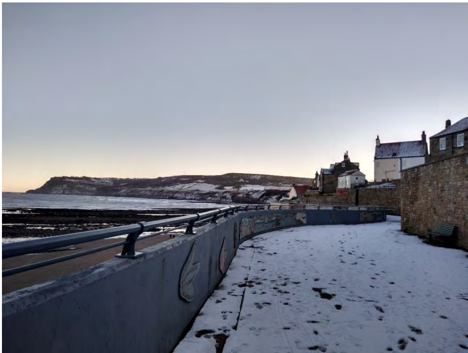
10 View looking south along sea wall. No vehicle access.
