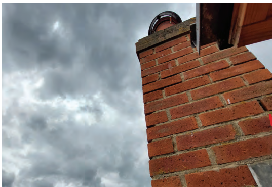
Modern chimney (a rebuild)
