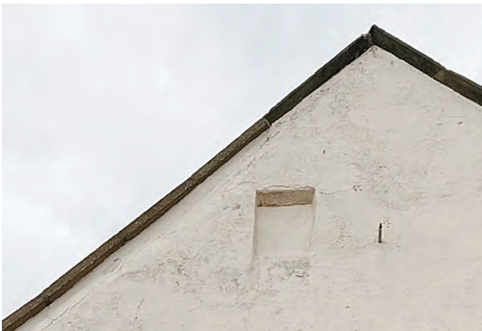
Blocked window to the rear
