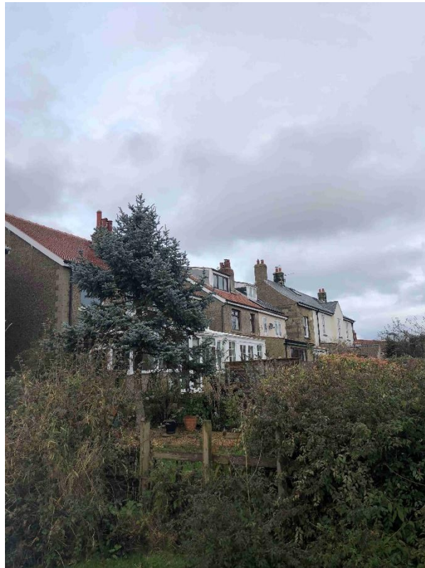
Photo 6 Rear elevation of the row
