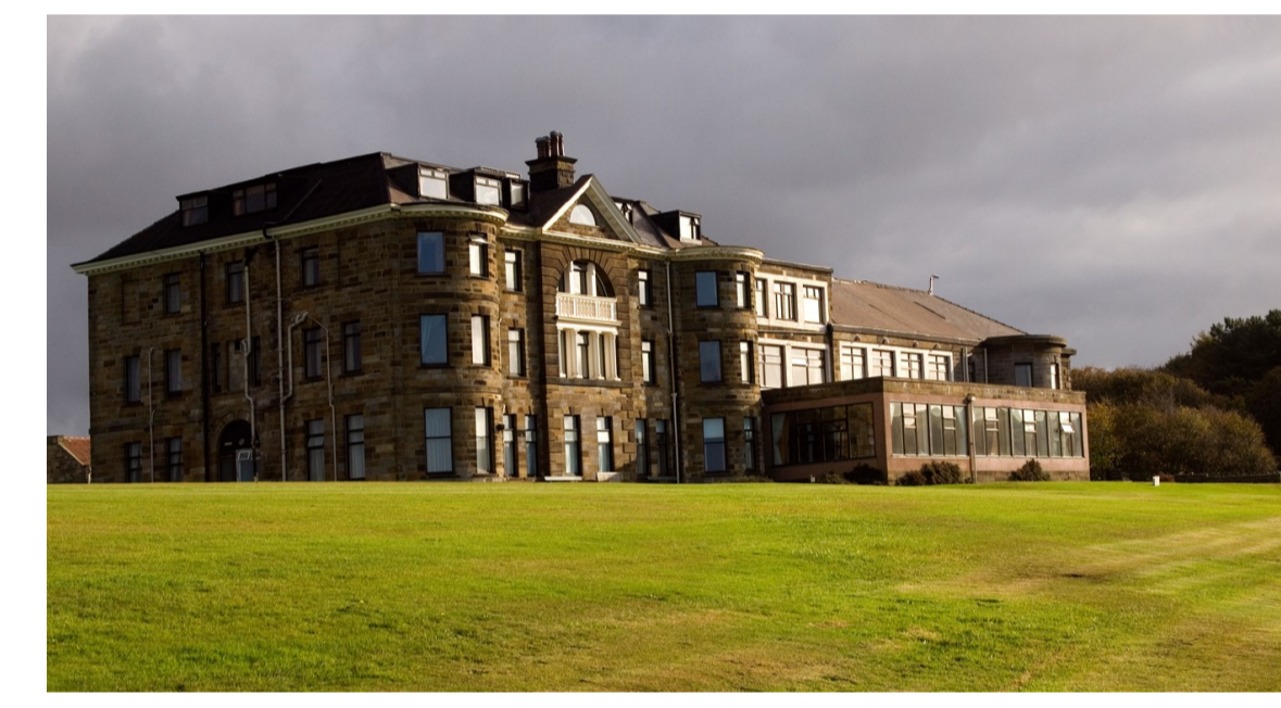
Photograph As Existing
