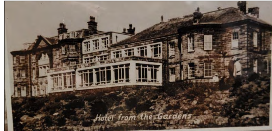
Figure 10 1938 Art Deco addition to the west
