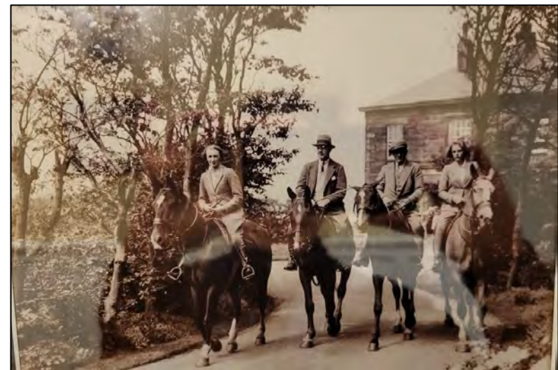
Figure 7 The east entrance to Raven Hall
