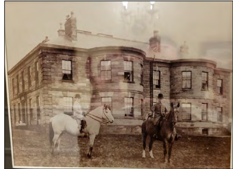
Figure 6 The original Raven Hall pre-1895
