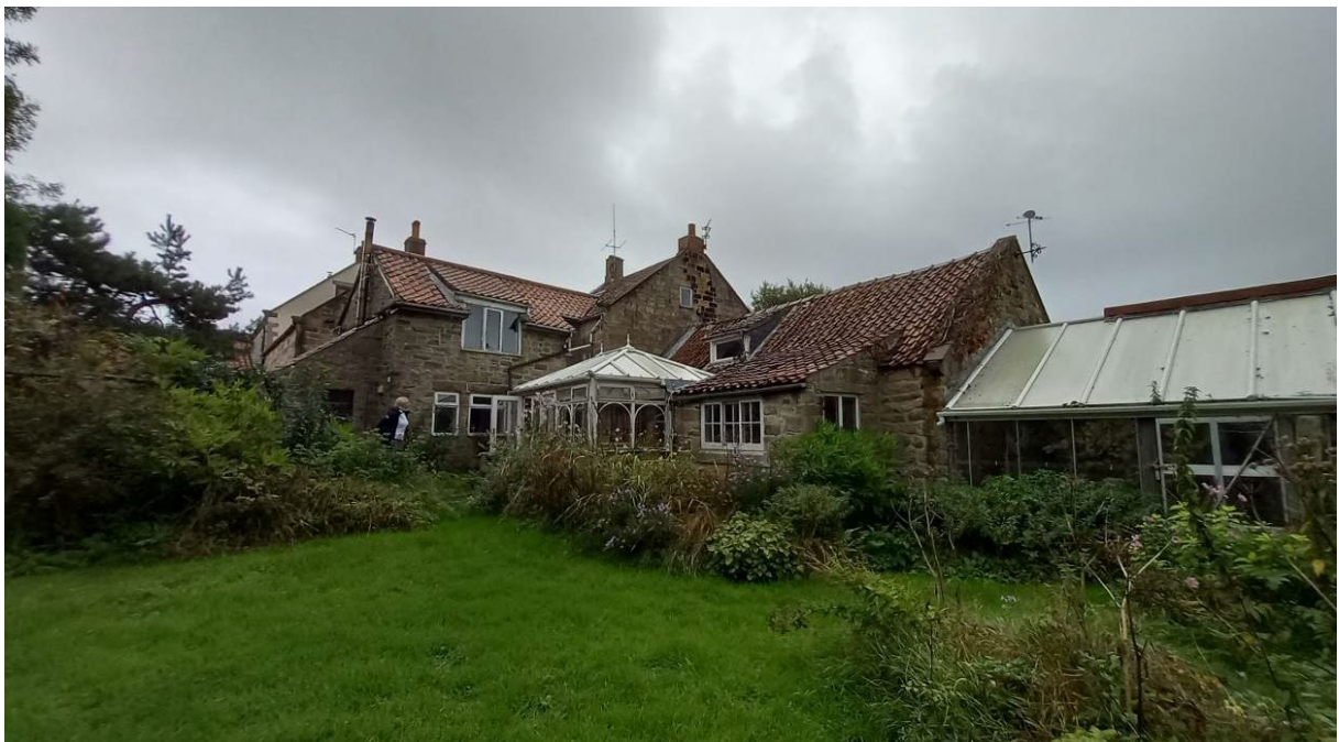
Photo showing the rear elevation of the dwelling.
