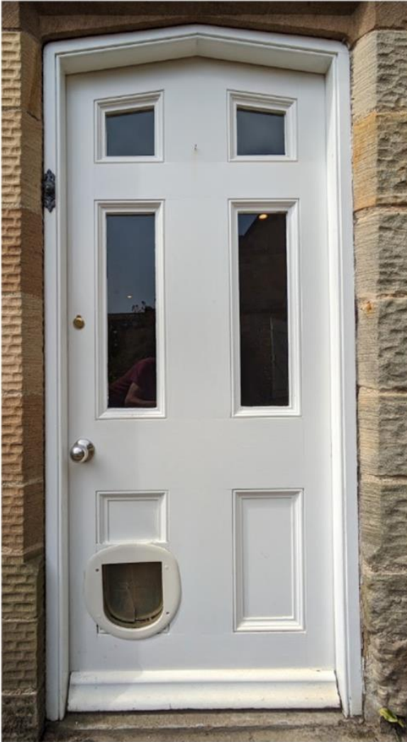
Existing kitchen door
