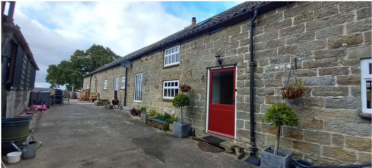
Photo of Long Barn – prior to current works
