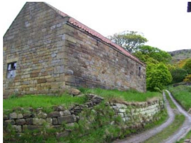
north and west elevations from access lane
