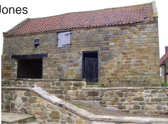
outbuilding east elevation from courtyard
