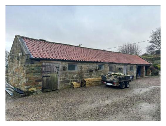
Photograph showing rear elevation of existing outbuilding proposed to be converted; air source heat pump and timber lean-to store also proposed to be constructed on this elevation.
