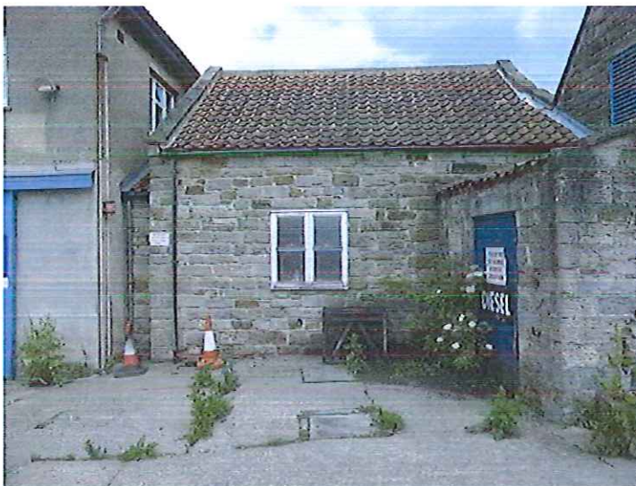
Plate 8 western elevation of building 3 with the stone facing
