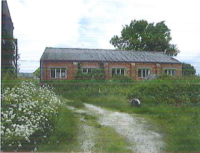
Plate 1 Building 1 viewed from the south looking north
