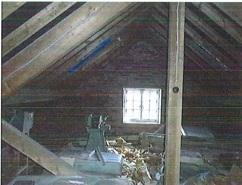
Plate 6 Roof void above the living accommodation within building 2
