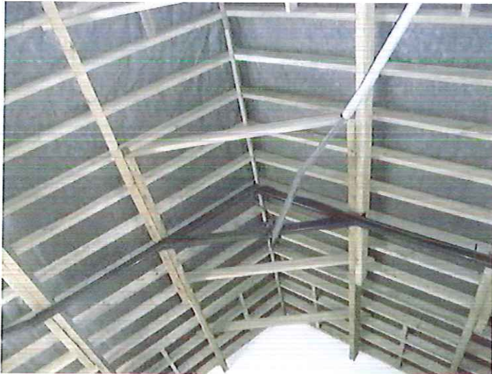
Plate 9 Internal view of the roof structure.
