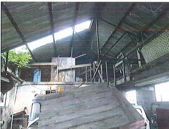
Plate 2 internal view of the roof structure
