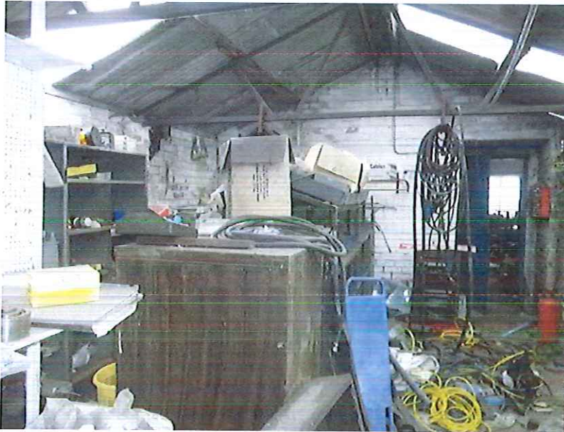
Plate 12 Internal view of building 4
