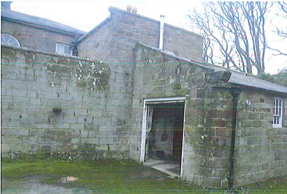
3.4 Park Hall North Elevation
