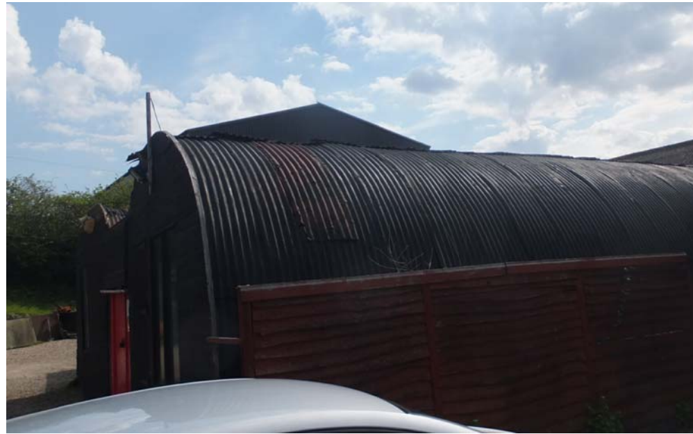
Example of Existing Nissen Buildings Onsite
