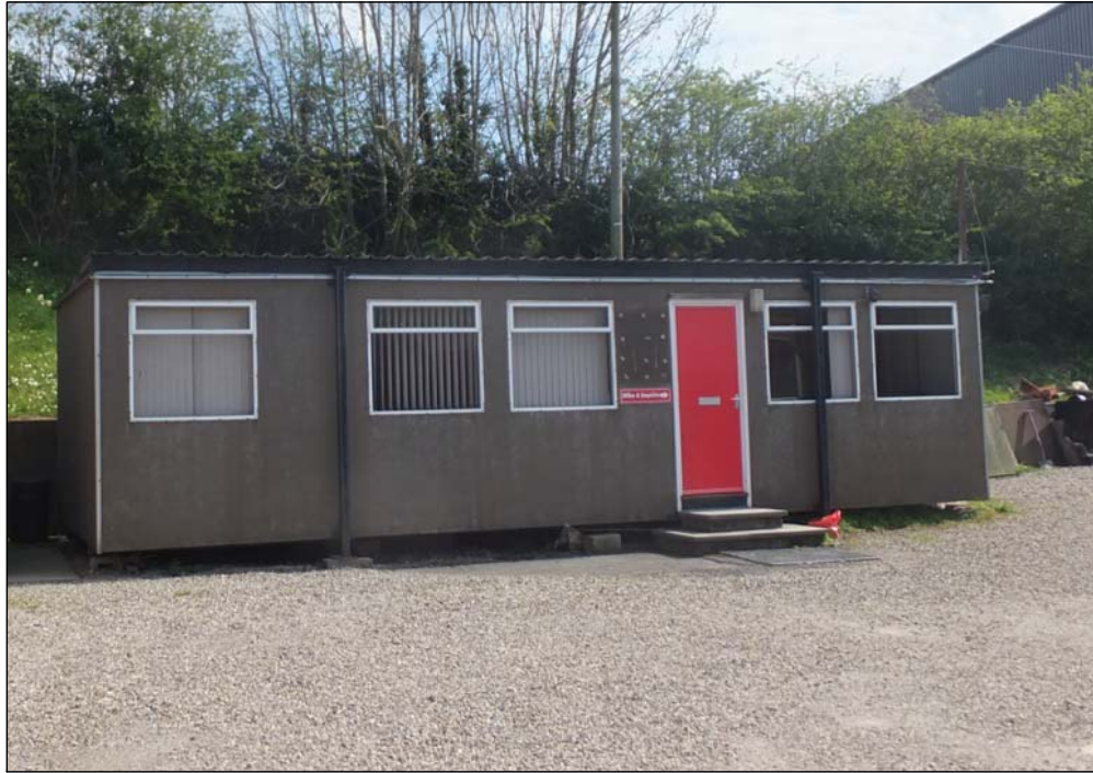
Existing Office Cabin (to be removed)
