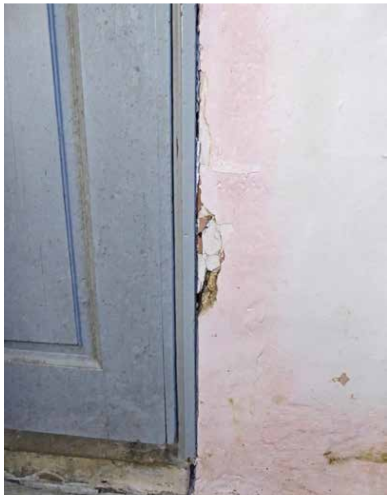
Chancel north wall. Plaster has failed to the side of the vestry door, on the east side a gypsum plaster repair has previously been carried out and this is now failing.
