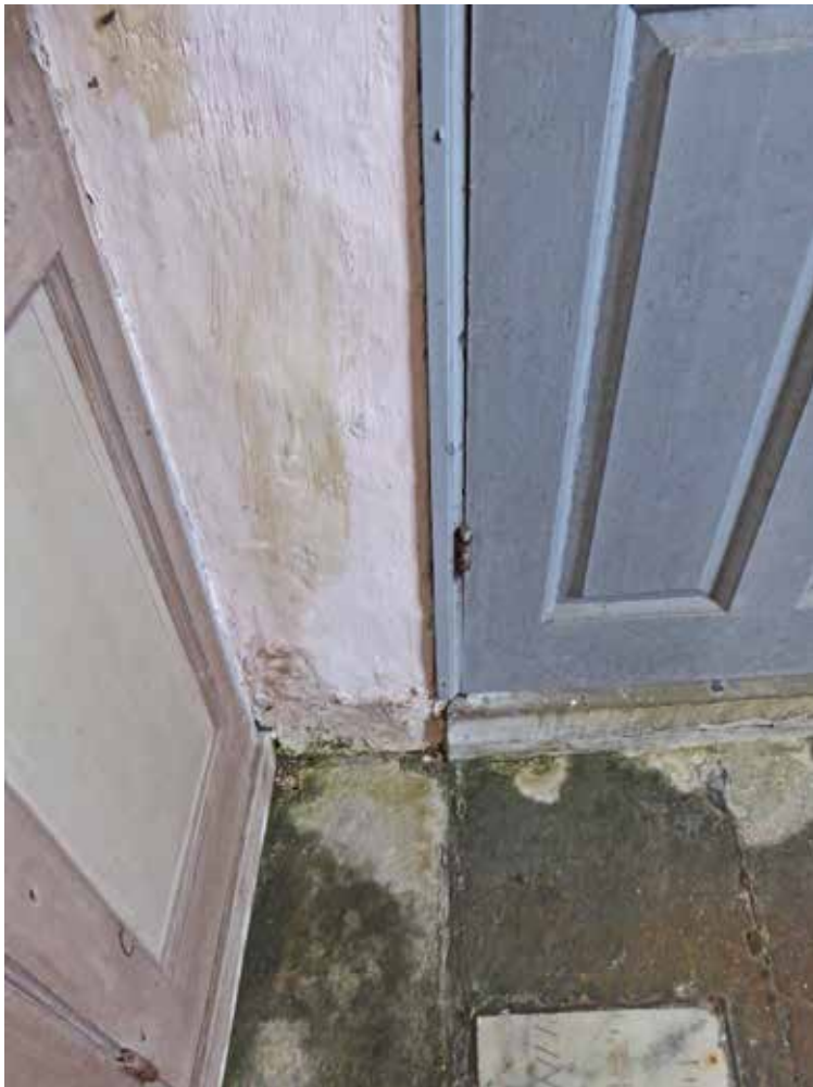
Chancel north wall. Plaster has failed to the side of the vestry door, on the east side a gypsum plaster repair has previously been carried out and this is now failing.
