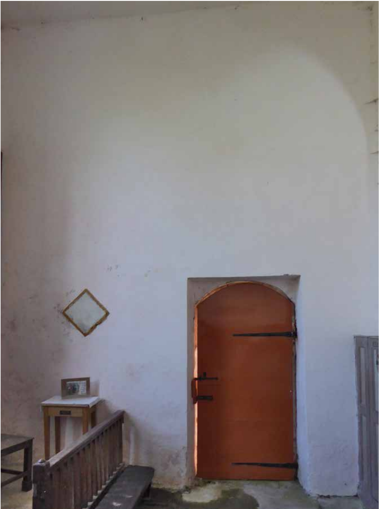
Chancel south wall.
