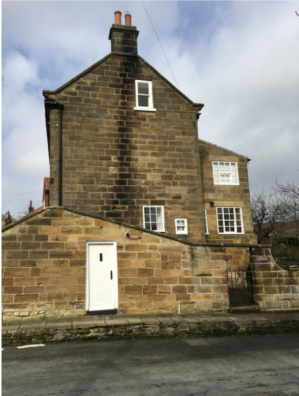
Photo 3 Side Elevation (East)
