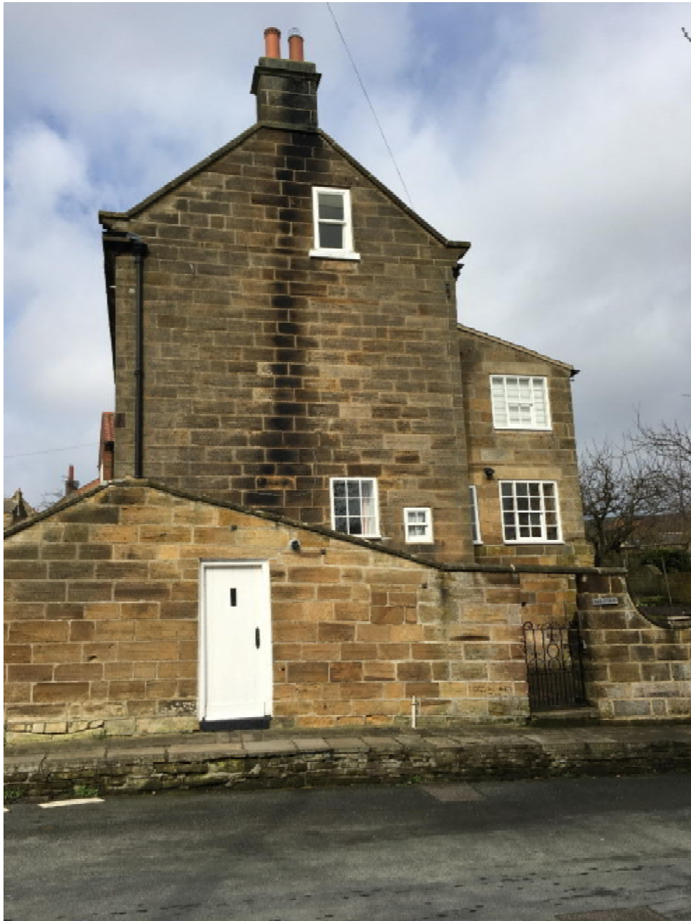
Photo 3 Side Elevation (East)
