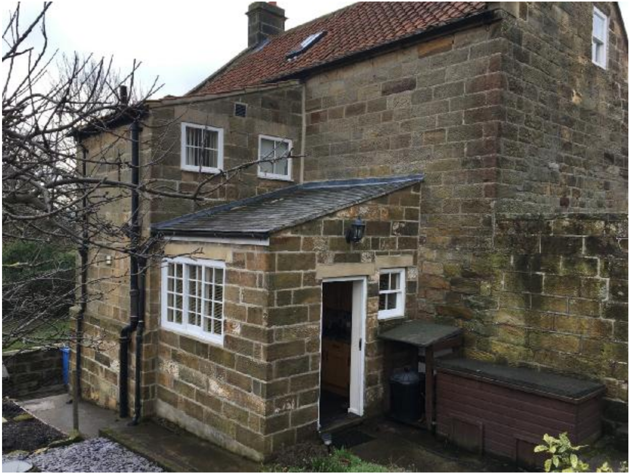
Photo 1 Rear Elevation showing Mono Pitch Extensions
