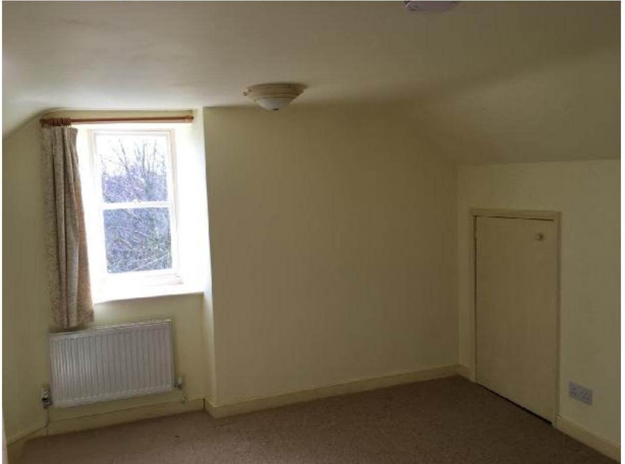
Photo 4 Stud Wall and Door, Attic Sitting Room
