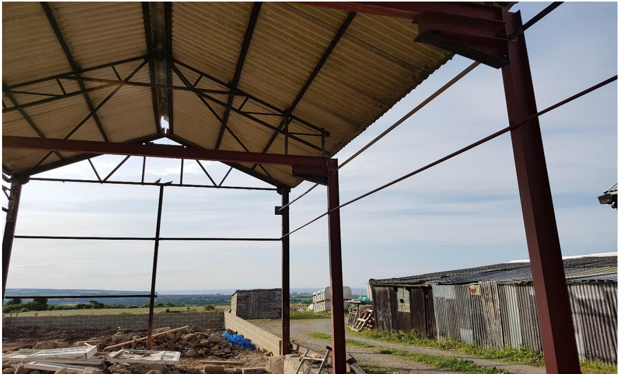
Figure 3. Evidence of existing steel frame
