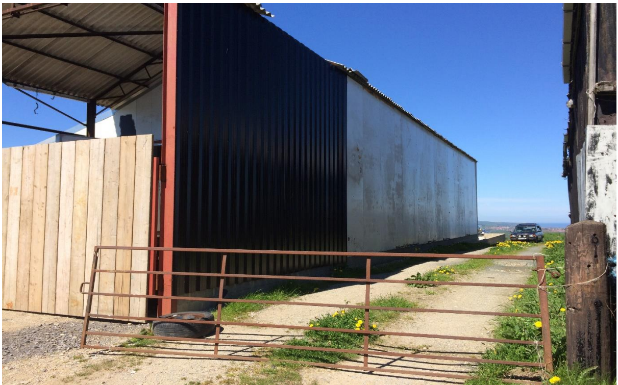
Figure 6. Shows dark coloured, like for like corrugated sheeting
