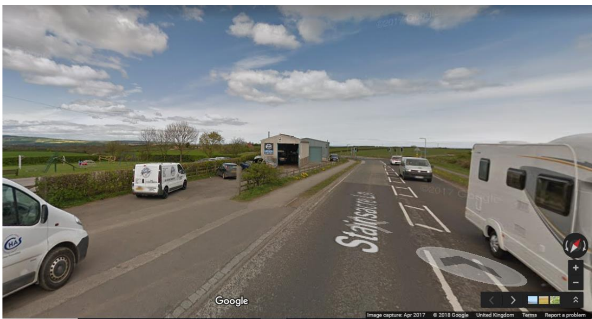
Figure 11. Bridge Garage, Hawsker
