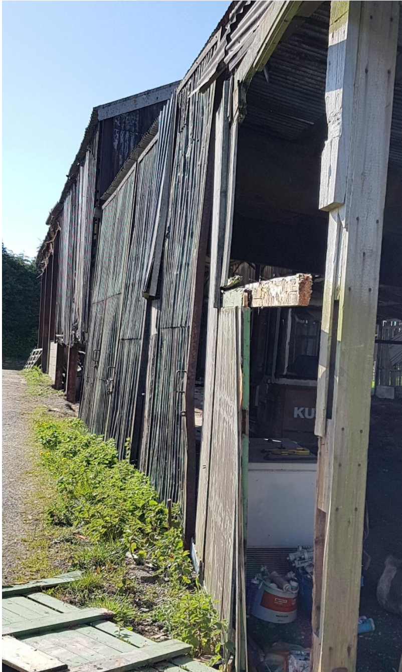
Figure 1. Original building prior to work commencing
