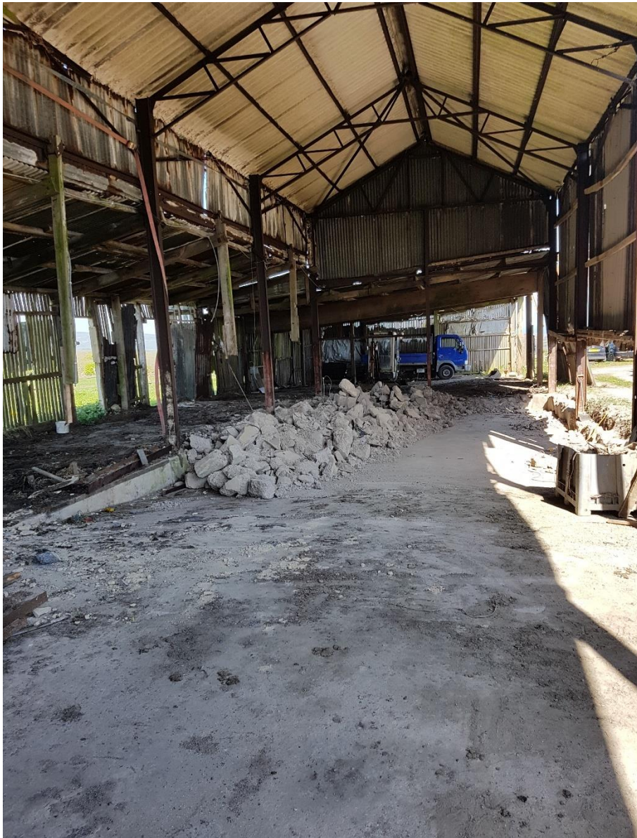
Figure 4. Main building showing frame, lean-to and stone floor
