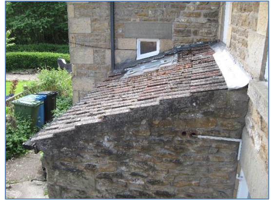
Photo 2: roof of extension
