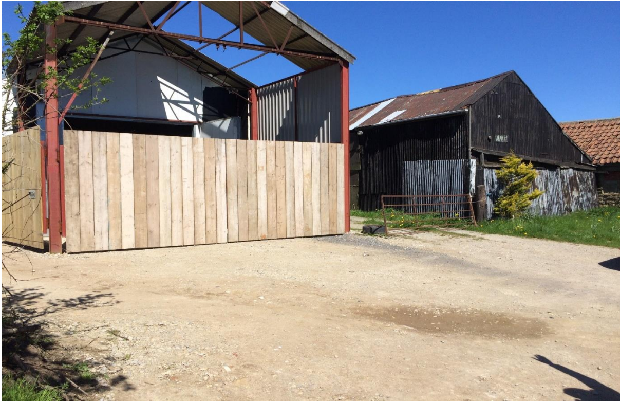
Figure 20. Photograph showing access apron to front of building – surface as existing – no works carried out.
