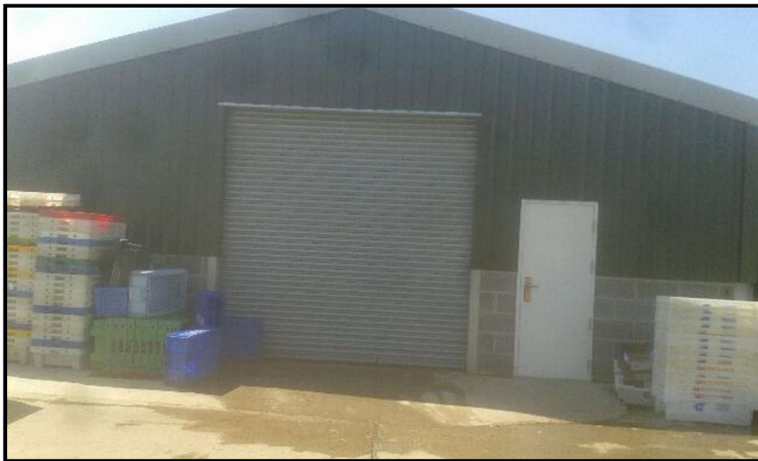
PHOTOGRAPH 1: EASTERN ELEVATION OF THE BUILDING
