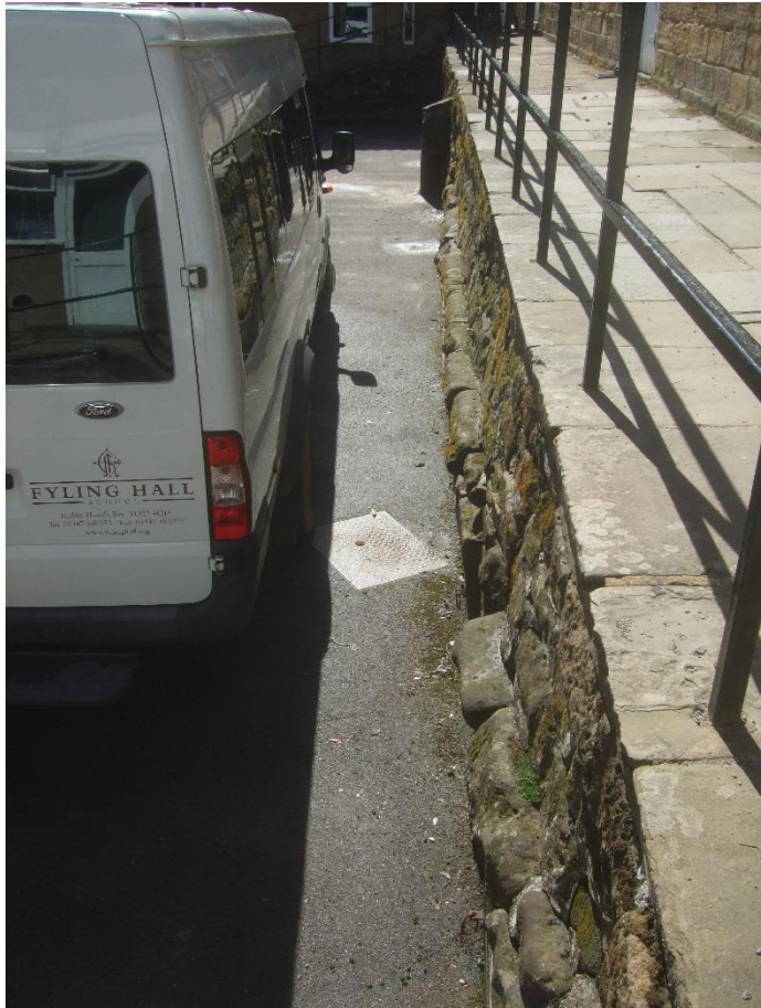
Photograph 2 – lower wall built in natural stone
