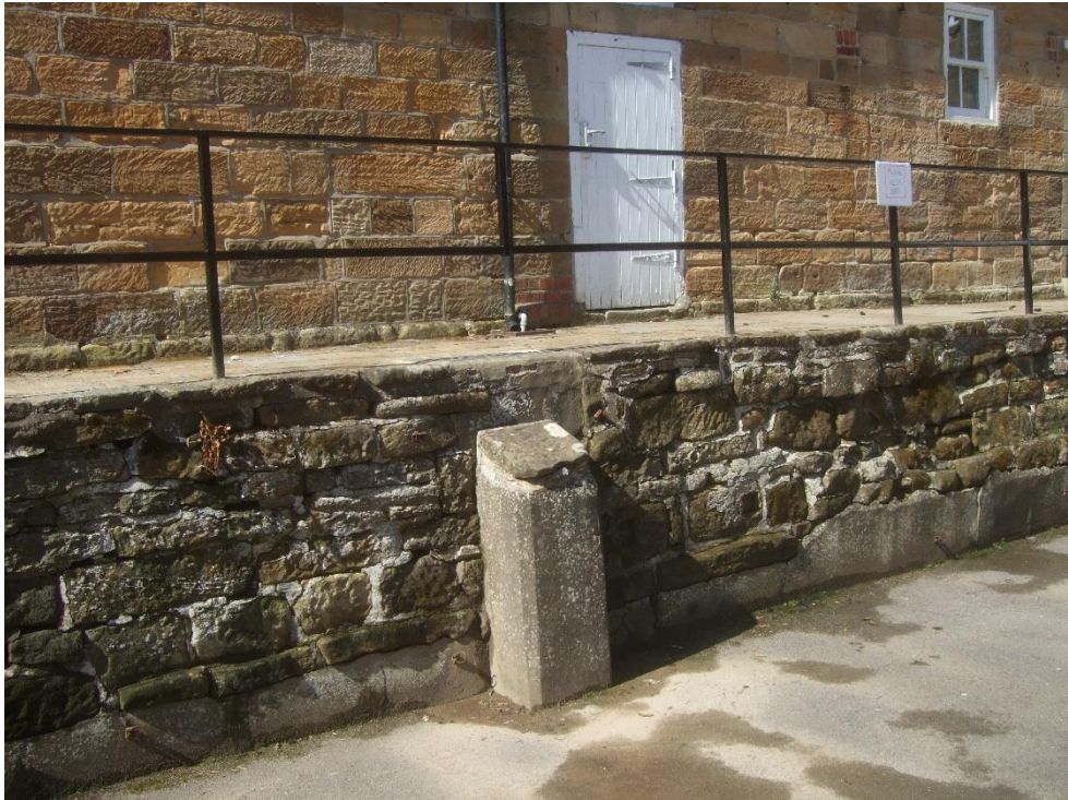
Photograph 6 - cover to vertical drain run(drain runs below the building)
