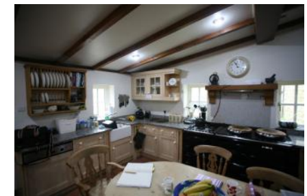
Fig. 12: Internal view of kitchen extension - proposed to be removed / replaced. Image shows low roof pitch and eaves height.
