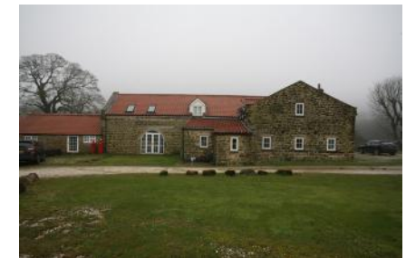
Fig. 9: View of the North elevation with lean-to kitchen elevation in the centre to be removed
