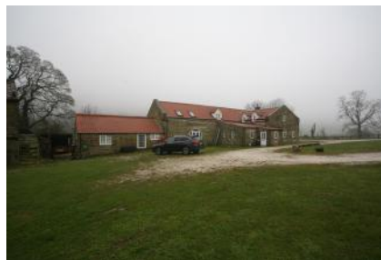
Fig. 10: View from garden of North elevation in a South West direction
