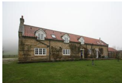
Fig. 7: View of South West / front elevation
