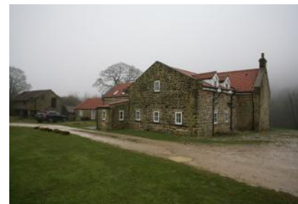
Fig. 11: View of rear / North West elevation of dwelling with agricultural buildings beyond
