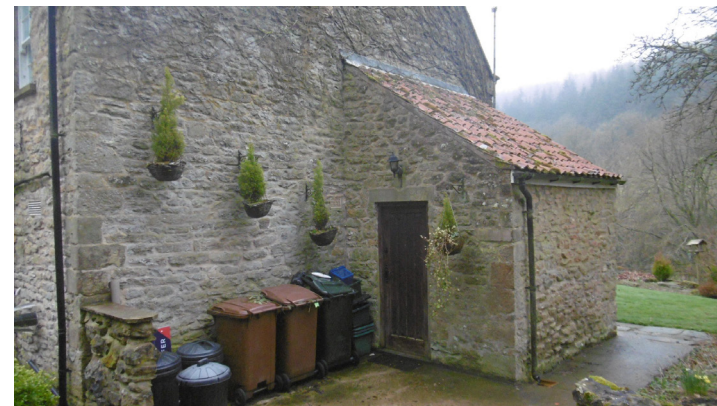
The above image shows the North elevation of the existing porch
