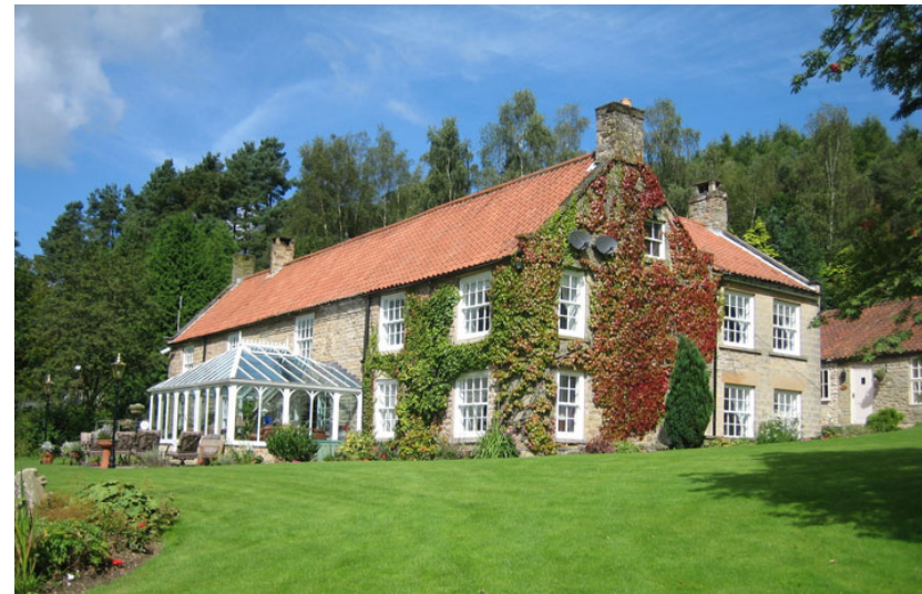
South elevation of the property constructed of stone with a pantile roof and a modern conservatory.
