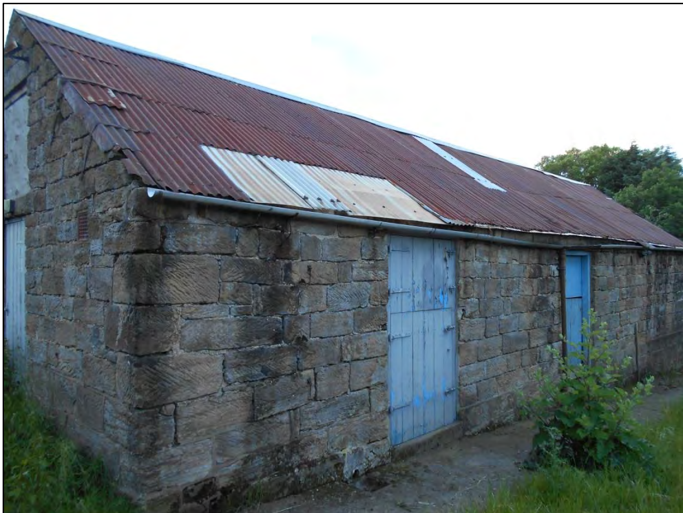
Figure 14: East side of building
