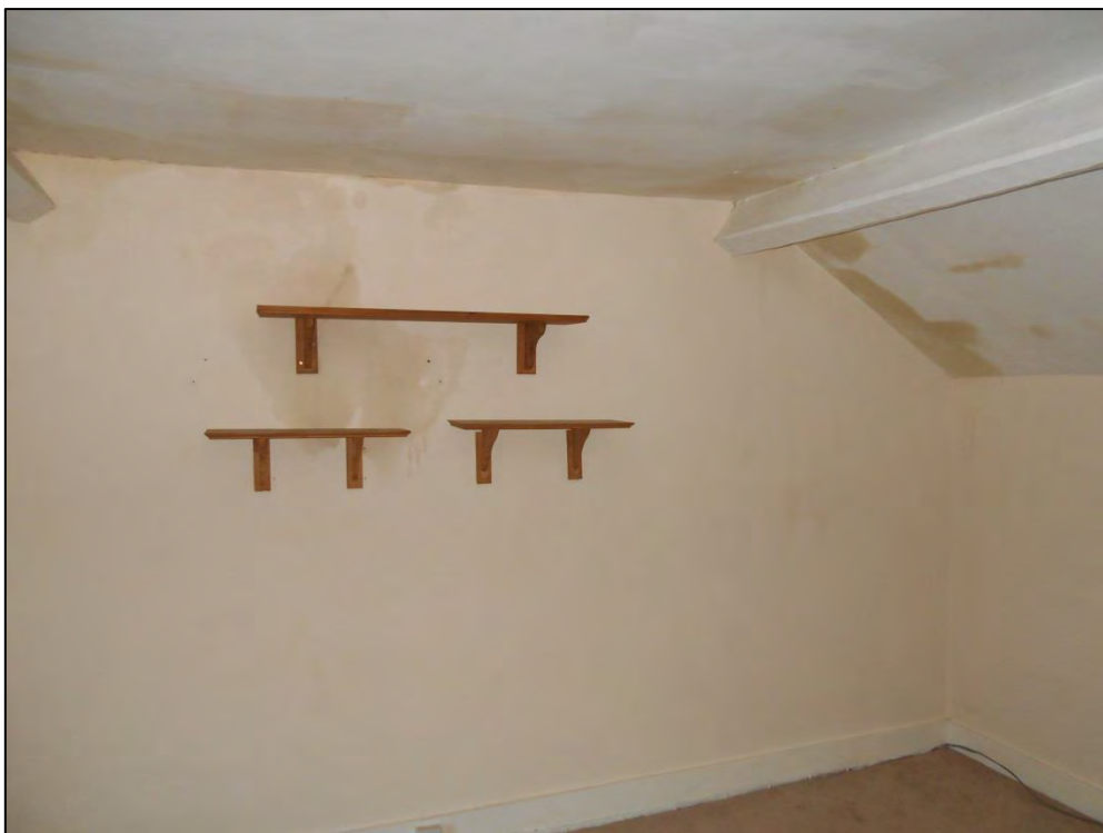
Figure 23: Interior of first floor of house showing absence of roof void
