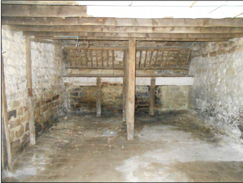
Figure 26: Interior of barns, central section
