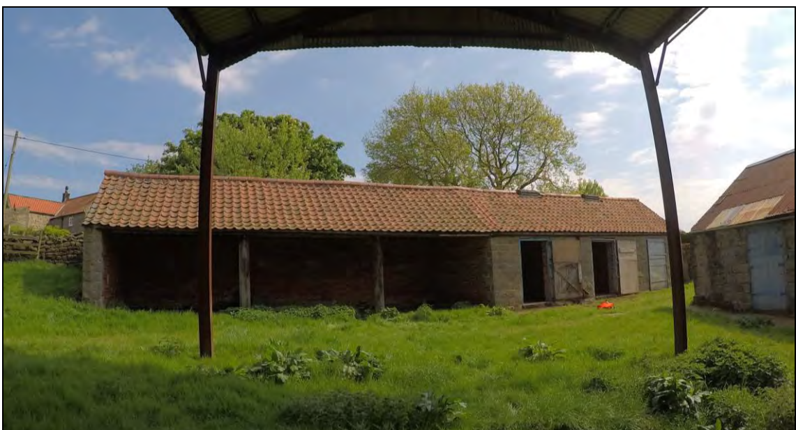
Figure 7: Existing photograph of Barn 2 front elevation / north side
