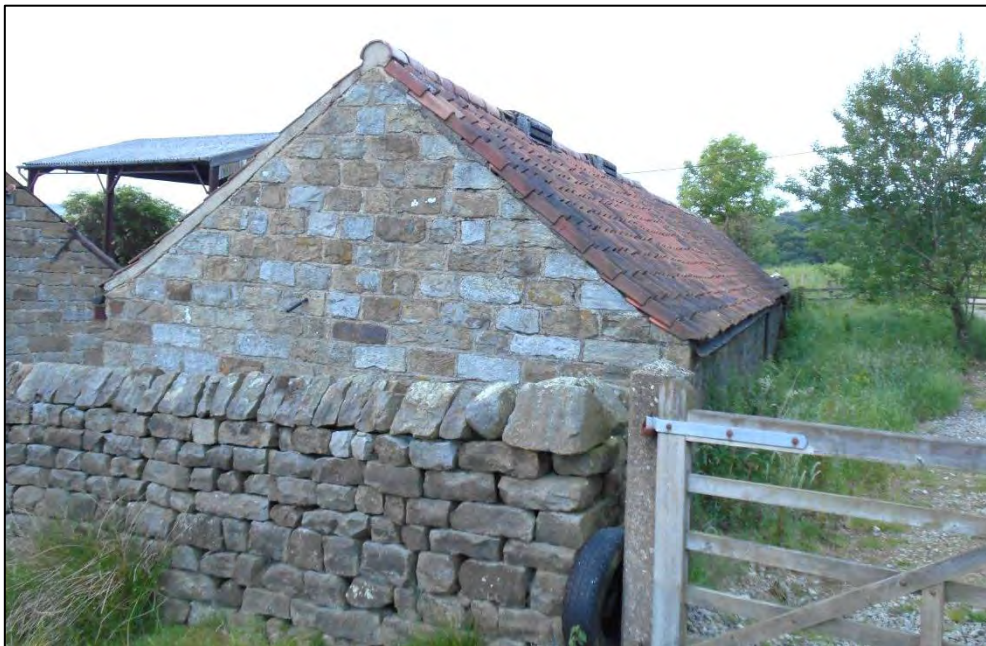
Figure 7: West end and south side
