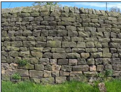
Figures 17 & 18: Existing drystone walls to corral to be retained; where wall is in deteriorated / partially collapsed state, wall to be reinstated, with some realignment as noted
