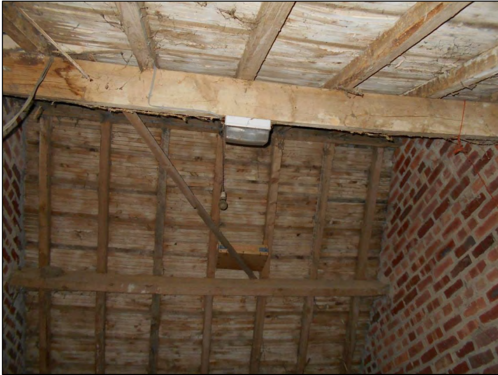
Figure 12: underside of roof of western section
