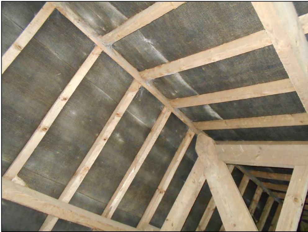
Figure 10: Underside of roof of eastern part of the building
