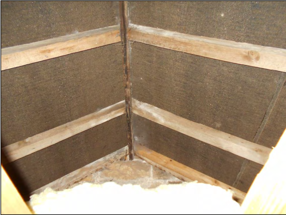
Figure 24: Underside of roof in small eastern house void
