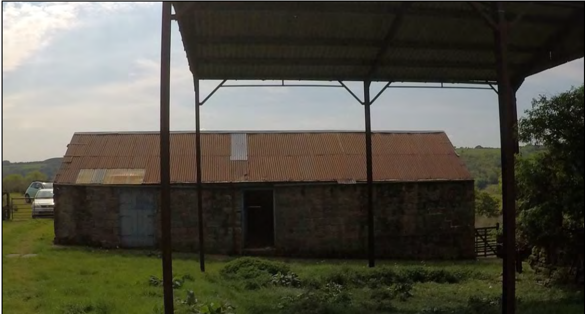
Figure 6: Existing photograph of Barn 1 front elevation / east side
