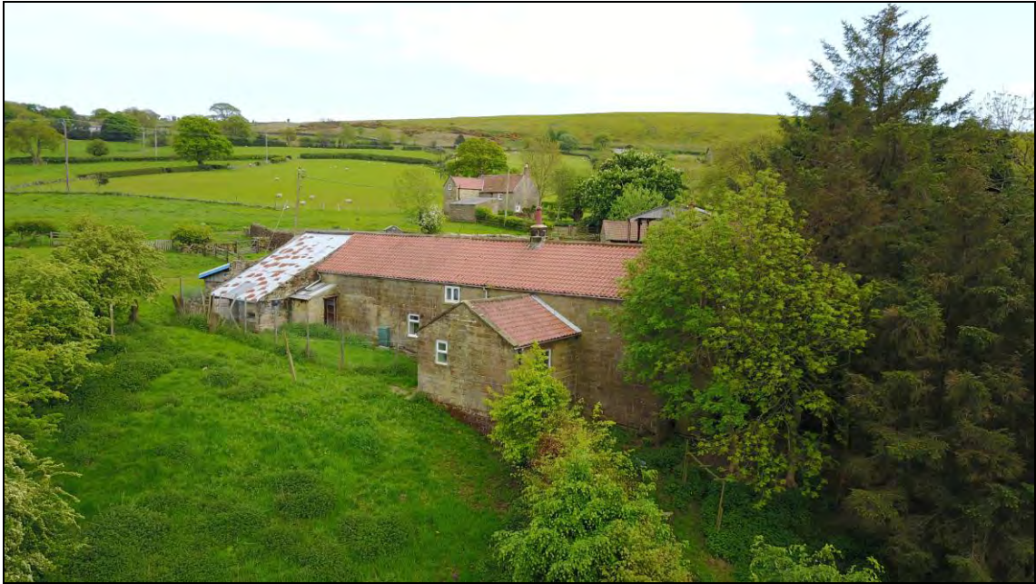
Figure 4: Existing aerial photograph of House, rear elevation / north side
