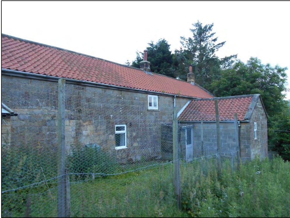
Figure 22: Western part of north elevation
