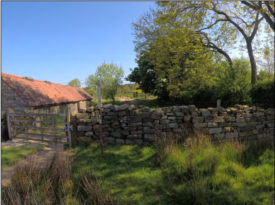
Figure 20: Existing gated access to south of Barn 2. Concrete post can be seen to left hand side; stone post to the right has cut, dressed face to right hand side, indicating it previously would have stood as the left hand post...furthermore, two stages of infill of a previous opening can be seen in the stonework to the right
