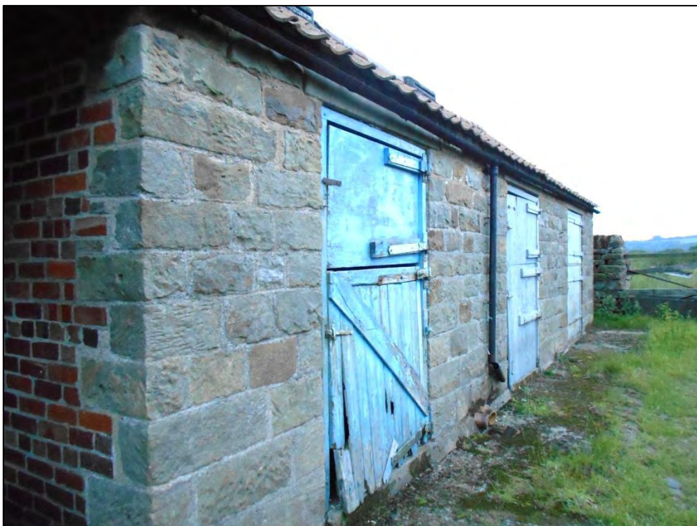
Figure 11: Western section, north side
