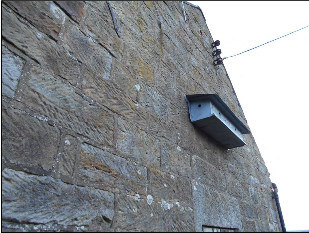
Figure 15: North gable end wall and sparrow terrace
