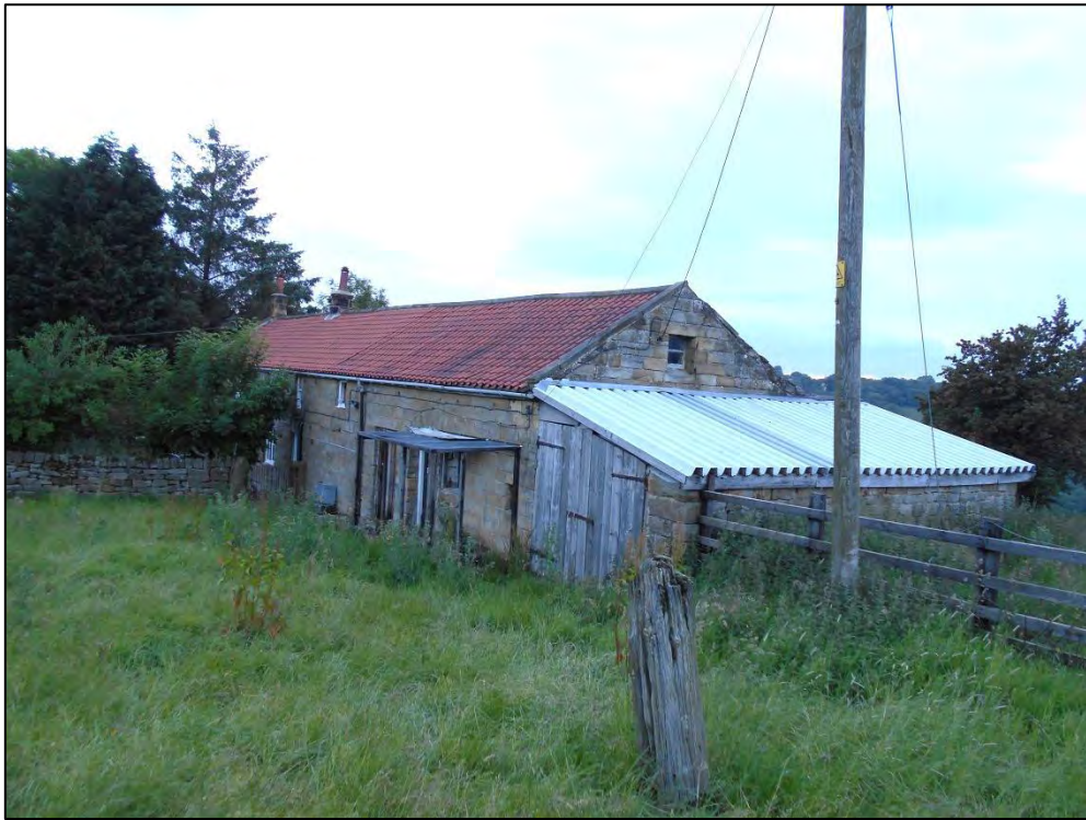
Figure 20: South side and east end
