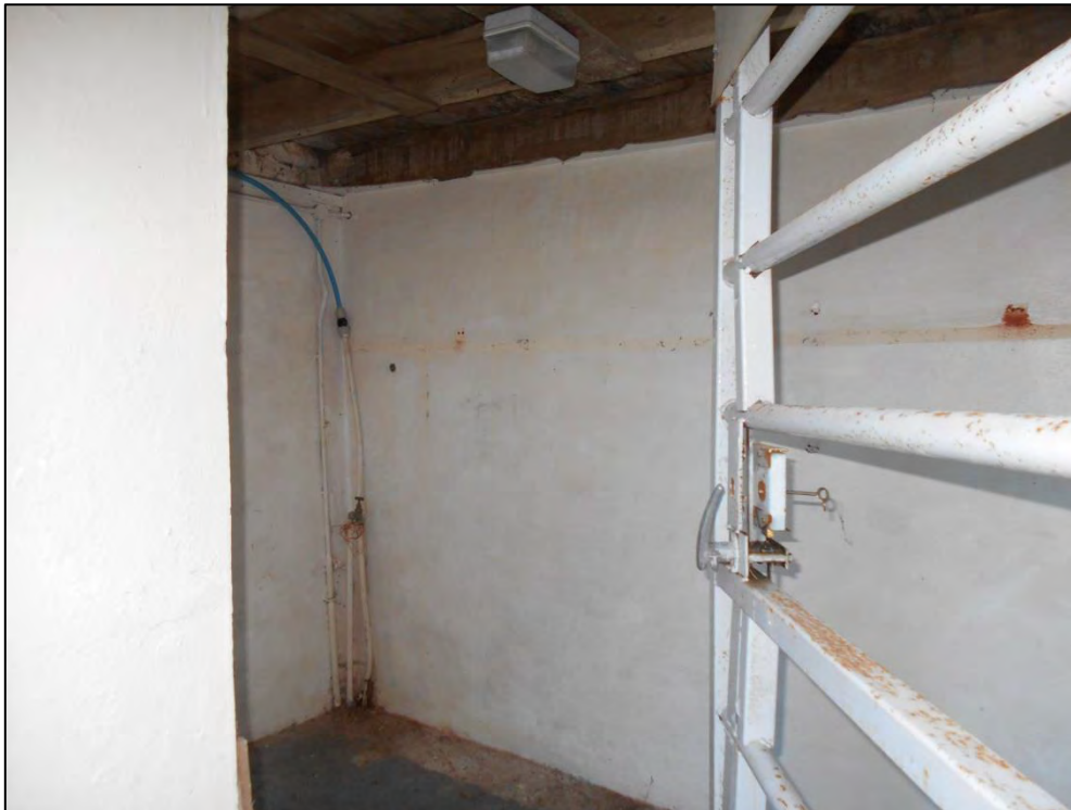
Figure 17: Interior of southern room
