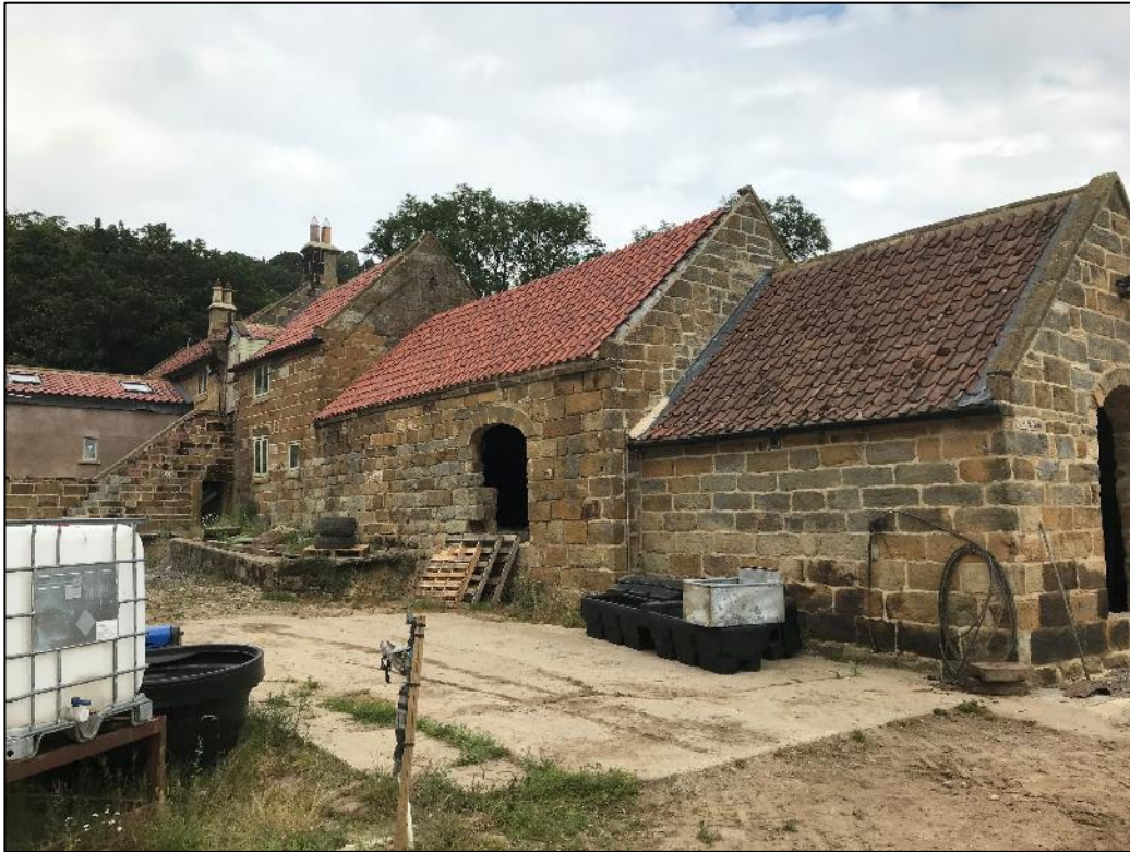
Photo 1 – View of rear of property
