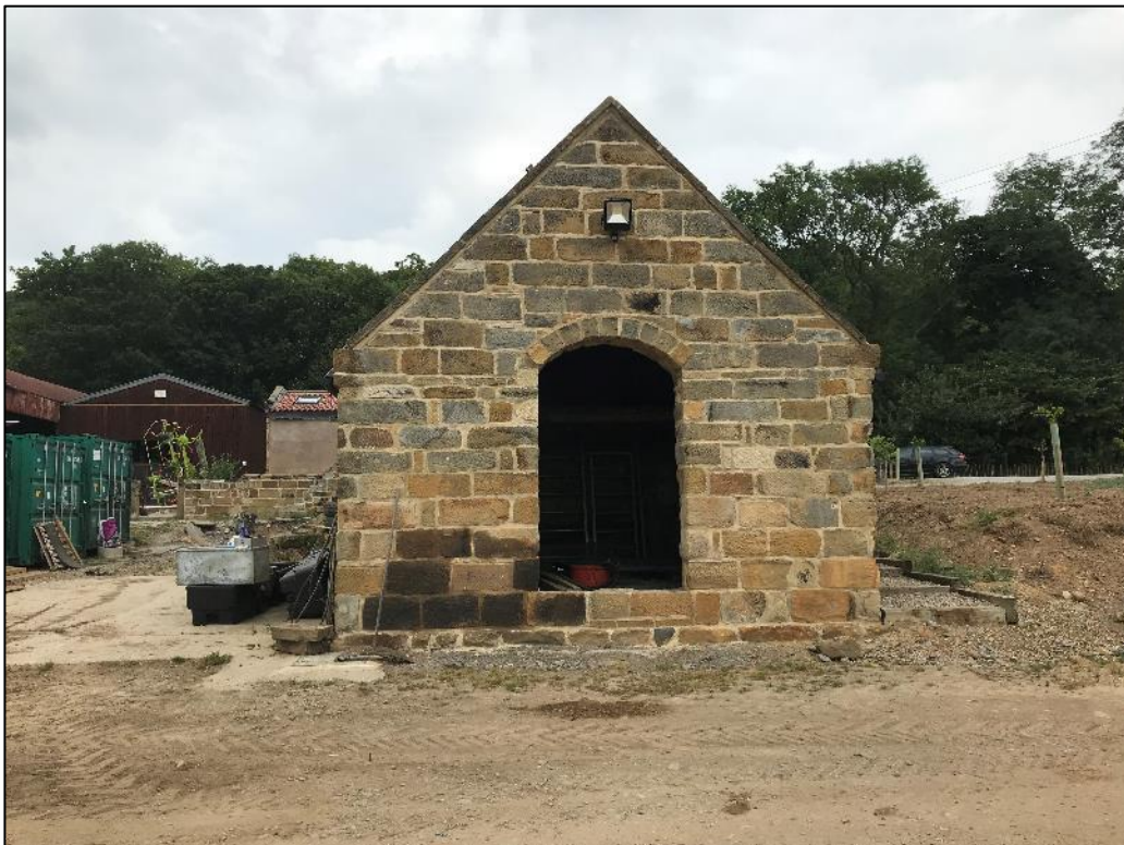
Photo 2 – View of side of property (including repaired/reinstated entry)
