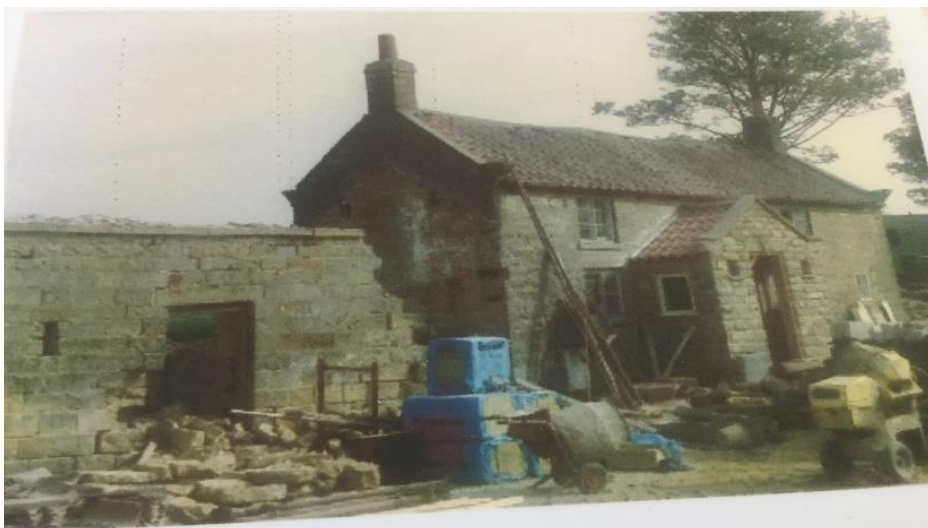
Fig. 6. Providence Heath, Cloughton – during construction – 1985 approx.
