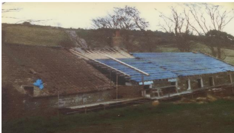
Fig. 8. Providence Heath, Cloughton – during construction – 1985 approx.
