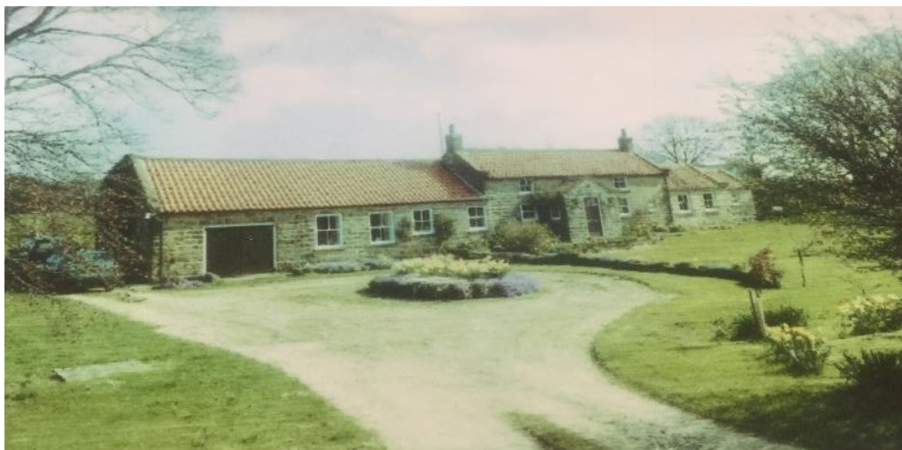
Fig. 10. Providence Heath, Cloughton – post construction – 1985/90 approx.
