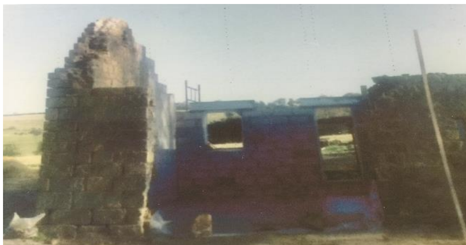
Fig. 9. Providence Heath, Cloughton – during construction – 1985 approx.
