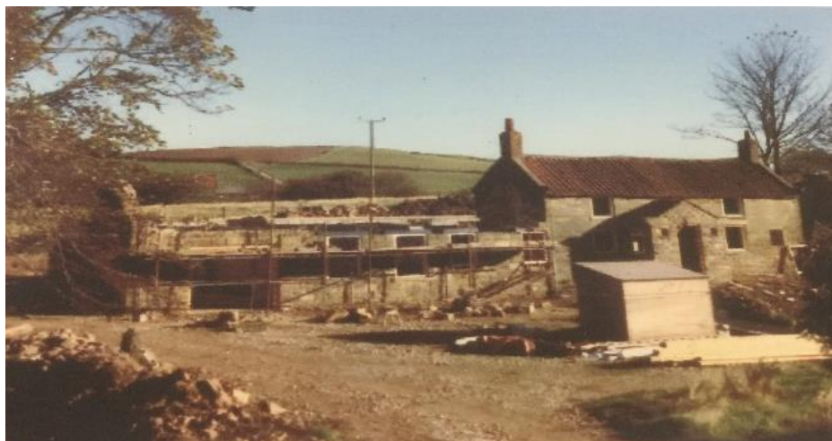
Fig. 7. Providence Heath, Cloughton – during construction – 1985 approx.
