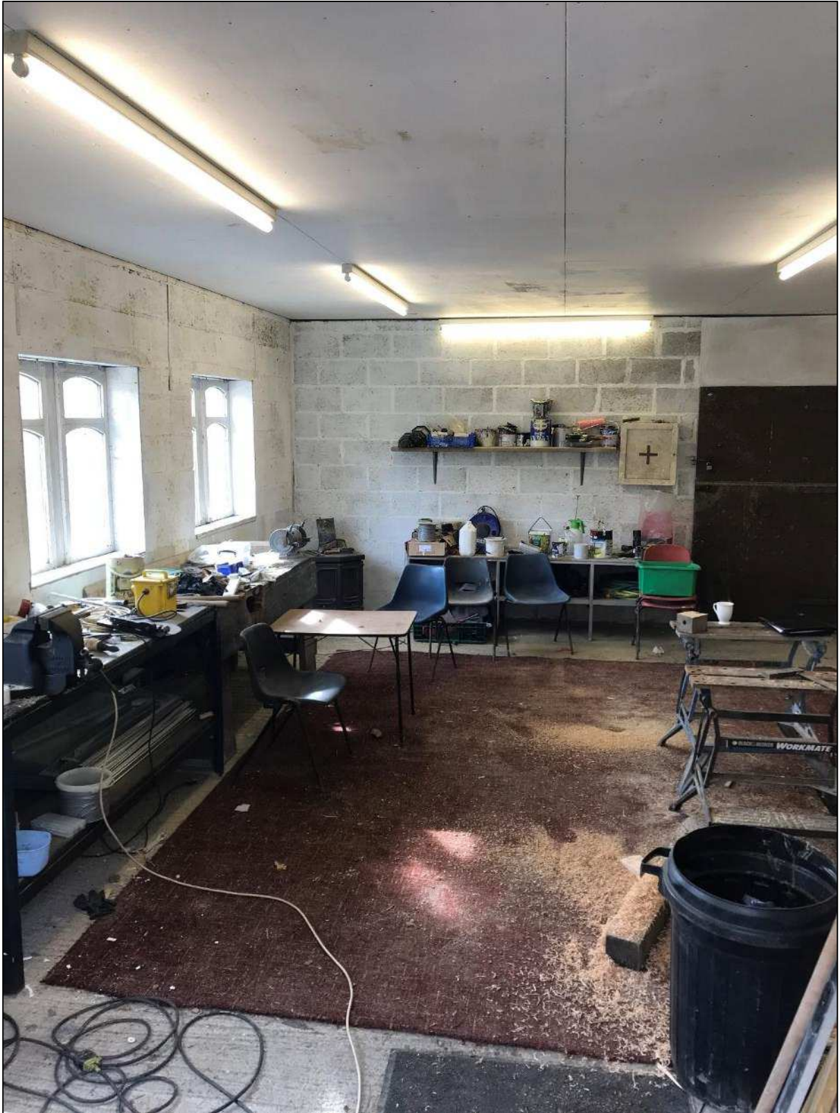
The room at the southern end of the building
