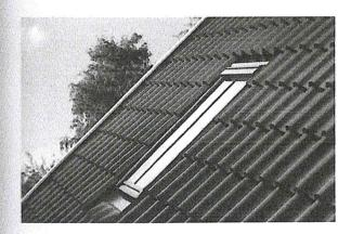
As well as the addition of a glazing bar, your local conservation officer may request that your roof window be installed deeper into the roof than can be achieved with a standard installation. To do this you should select a recessed flashing kit, which will provide a sleek, streamlined finish as less of the roof window protrudes above the roofline. Recessed flashings are also available with insulation and underfelt collars and are recommended for optimum energy efficiency.
