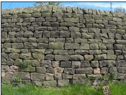
Figures 17 & 18: Existing drystone walls to corral to be retained; where wall is in deteriorated / partially collapsed state, wall to be reinstated, with some realignment as noted
