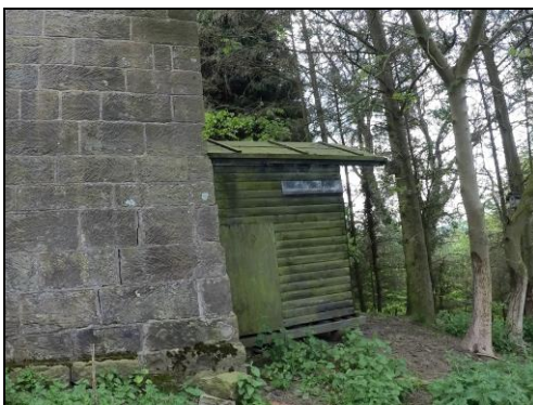
Figures 13 & 14: Evident subsidence to the north-west corner of the Main House, attributed to the extensive tree root systems of Larch and Leylandii trees in close proximity
