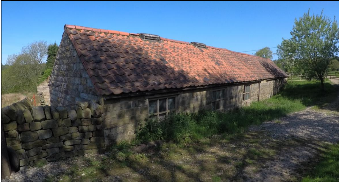
Figure 8: Existing photograph of Barn 2 rear elevation / south side (note: ground level built up against back wall and existing vehicular track passing towards proposed car parking corral beyond)
