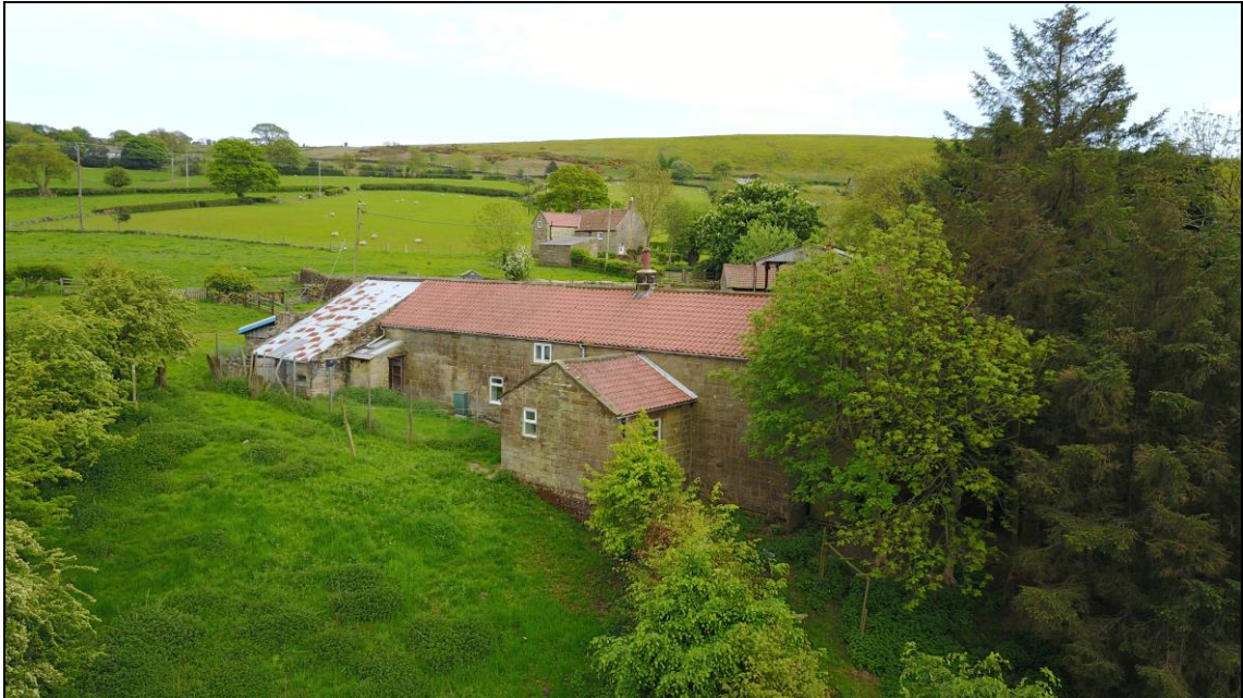
Figure 4: Existing aerial photograph of House, rear elevation / north side
