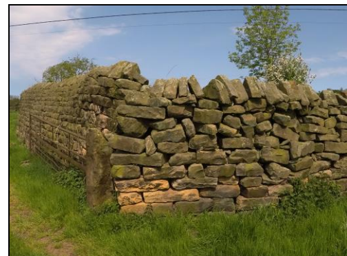
Figures 17 & 18: Existing drystone walls to corral to be retained; where wall is in deteriorated / partially collapsed state, wall to be reinstated, with some realignment as noted
