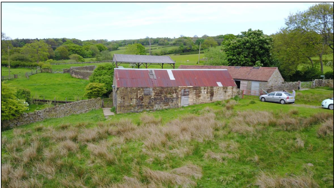
Figure 5: Existing aerial photograph of Barn 1, rear elevation / west side
