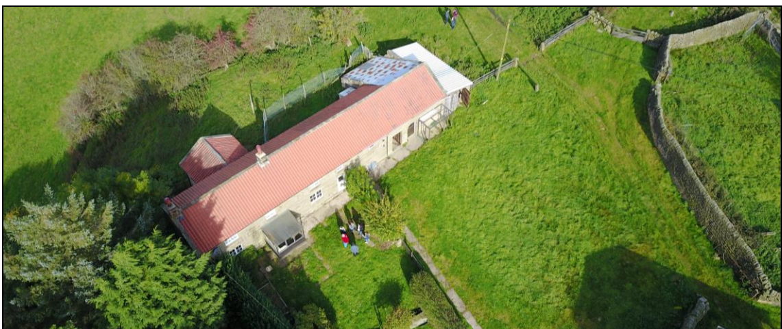
Figure 3: Existing aerial photograph of House, front elevation / south side
