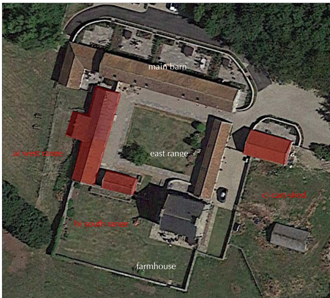
Figure 2: Google Earth aerial image showing the Thirley Cotes Farm complex with key elements annotated.
